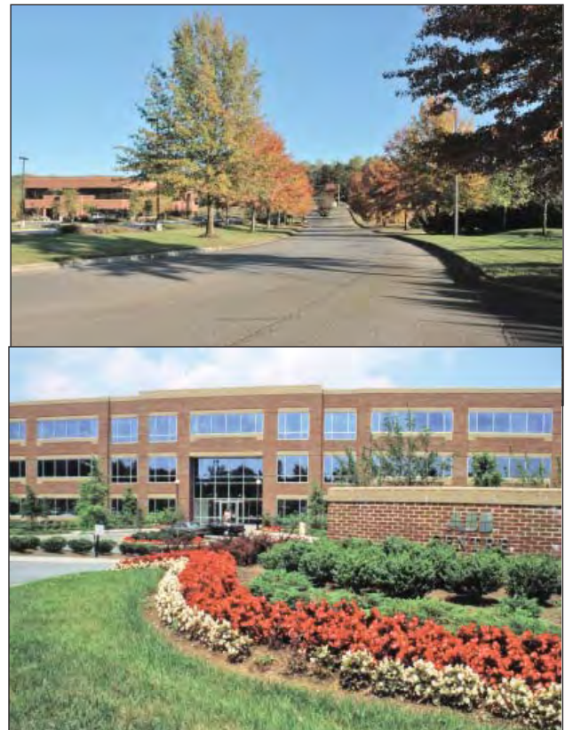
Above: Centerpoint Business Park has been the focus of significant office development.
