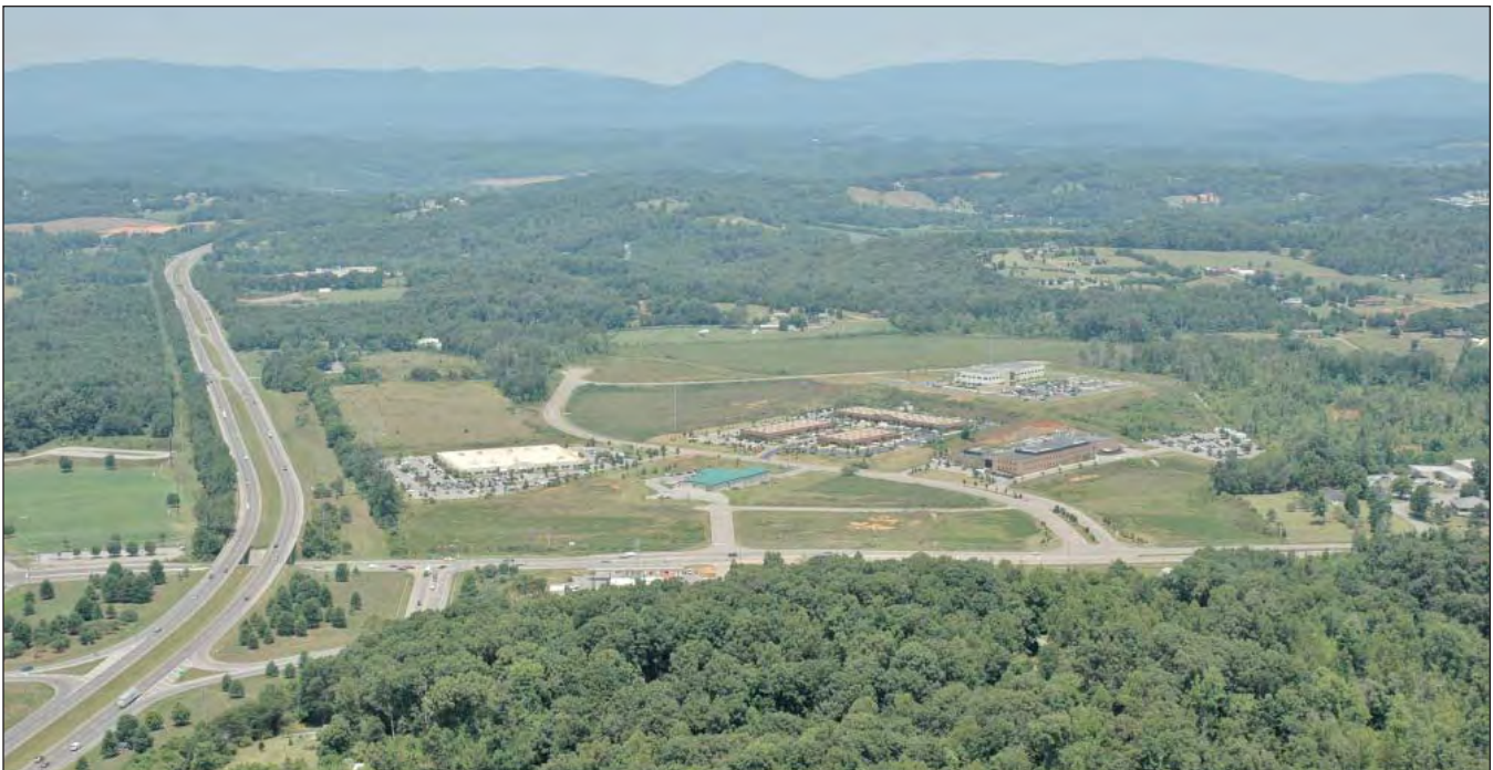
Below: An aerial view of Pellissippi Corporate Center in 2006
