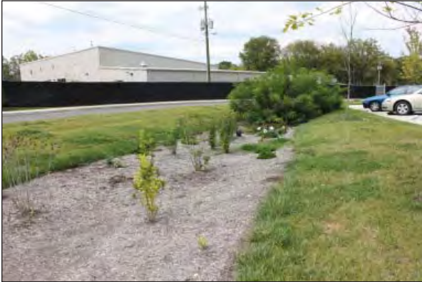
This bioretention swale is located at the Hallsdale-Powell Utility District headquarters.
