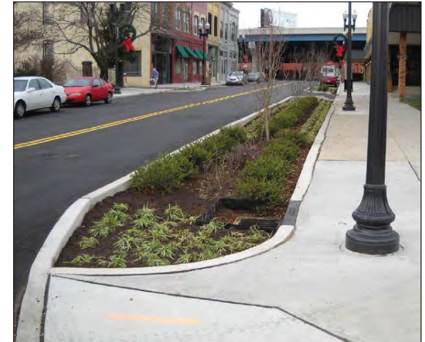
Streetscape improvements to N. Gay Street included new sidewalks, lighting, on-street parking, and landscaping with bio-retention to infiltrate stormwater runoff.
