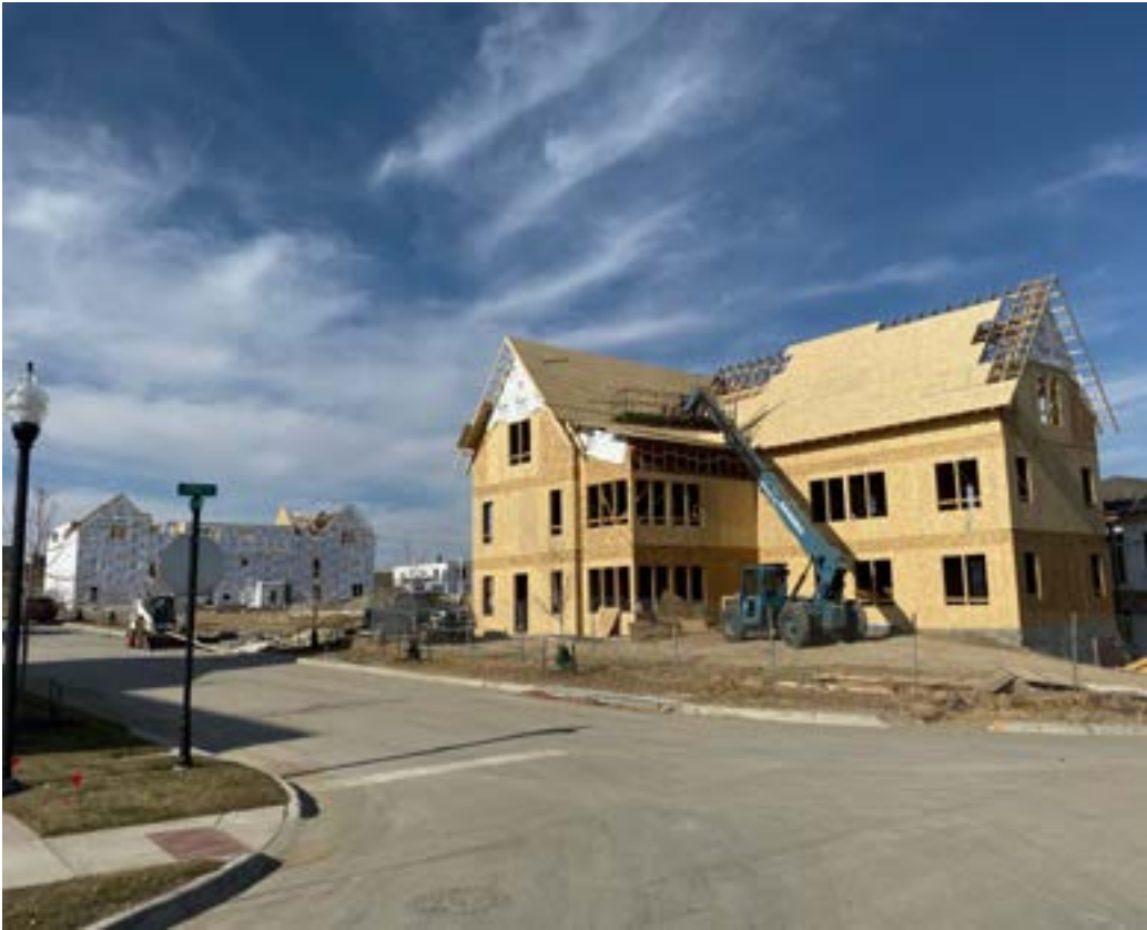
Figure 2.4 The simple forms, smaller size, and compatibility with wood-frame construction help maximize affordability and investment returns, and are consistent with the construction strategies familiar to most residential homebuilders, as shown in this under-construction MMH project in Papillion, Nebraska.
