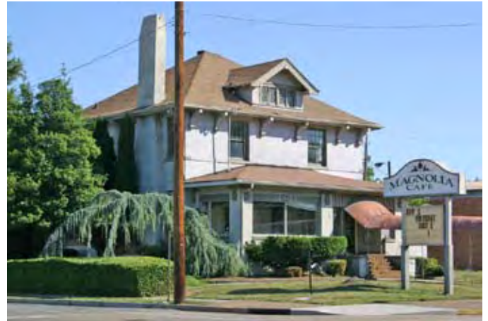
One of several early 20th Century houses that have been converted into commercial property.
