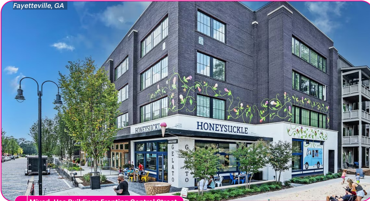
Mixed-Use Buildings Fronting Central Street
