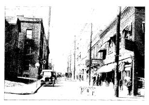
Poles and Wires on Market Street. The overhead wires and wooden poles mar the appearance of this block on Market Street. Note the improved appearance of the street where wires have been placed underground.
