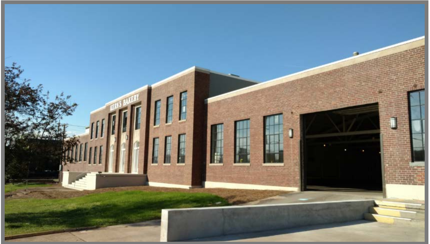
The former Kerns Bakery building front façade as seen from Chapman Highway.
