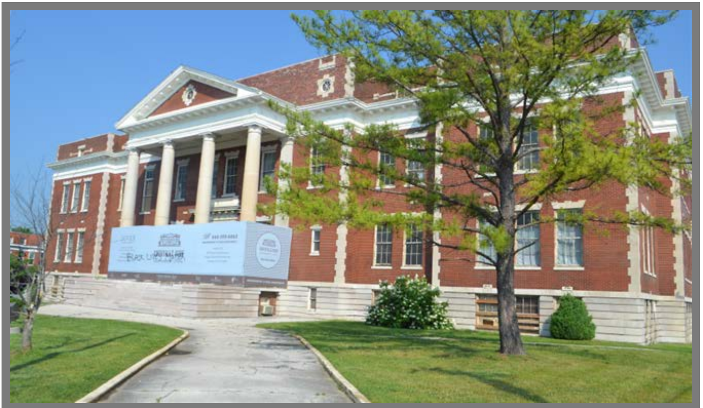
Historic Knoxville High School 2016 – pre-renovation
