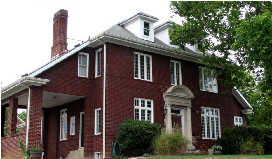
1803 Clinch Ave. Front Facade
