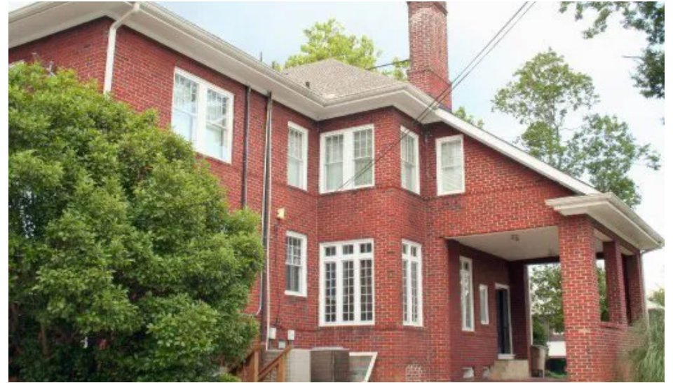
1803 Clinch Ave. West Facade
