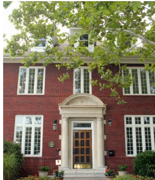
1803 Clinch Ave. Entry
