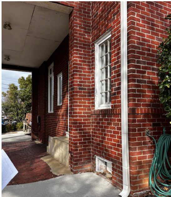
1803 Clinch Ave. Carriage Porch
