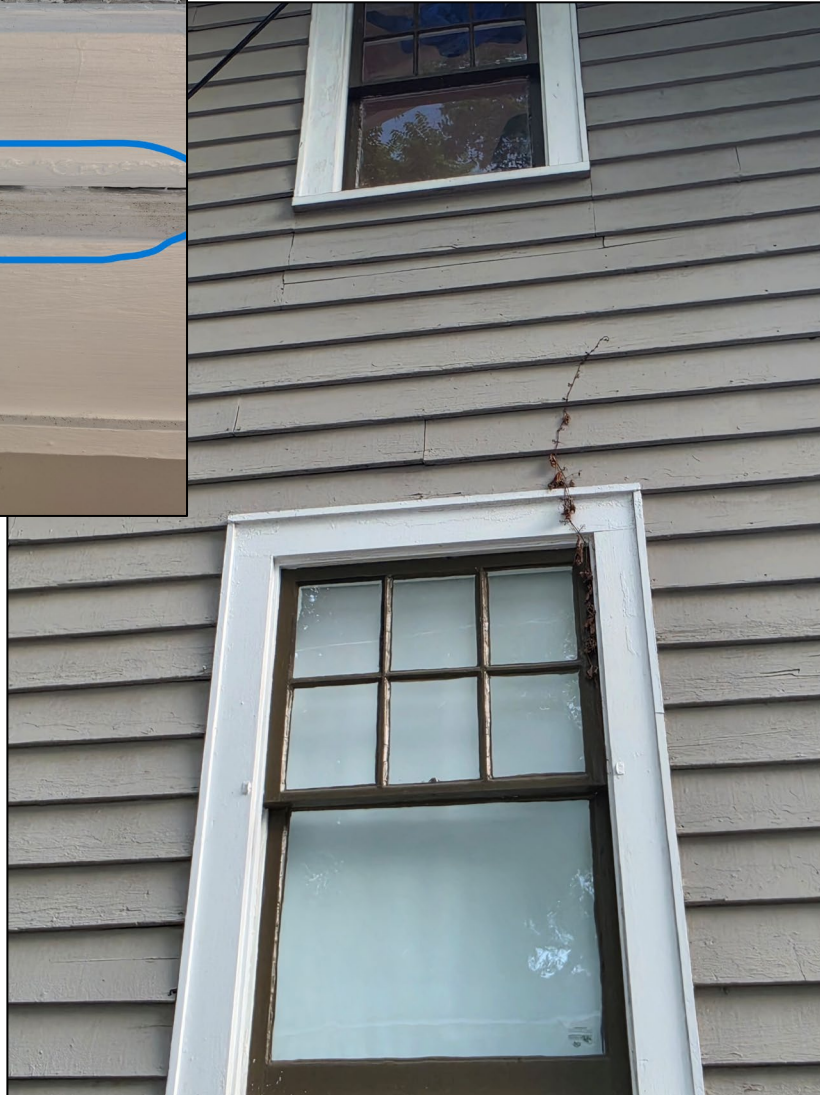
Downstairs bathroom, exterior
