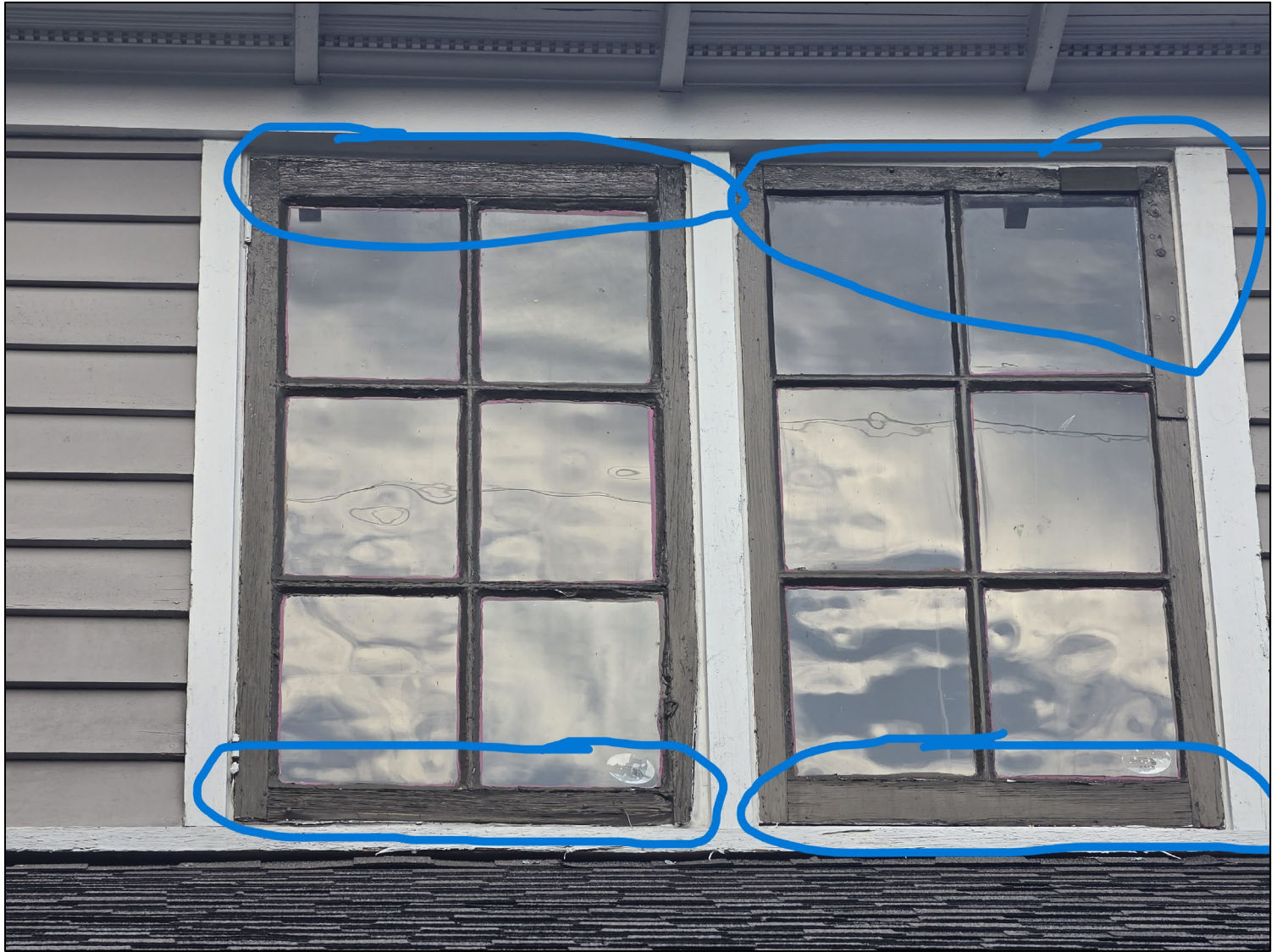
Upstairs bedroom exterior
