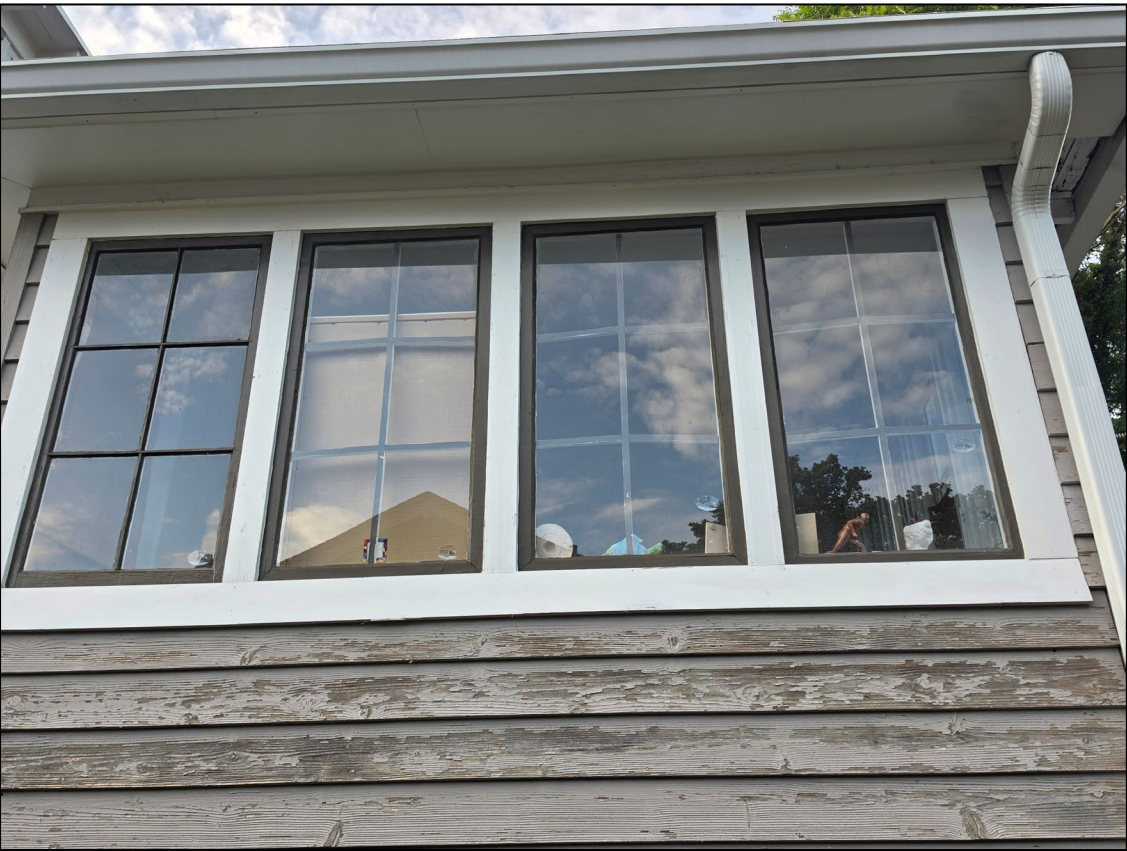
Three non-historic windows in office (south elevation)
