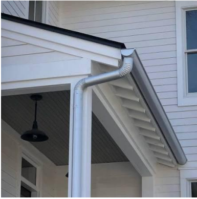
Half-round gutters: galvanized
