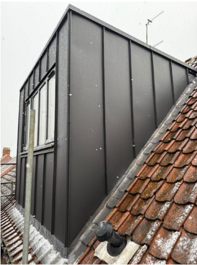
Dormer w/ zinc cladding
