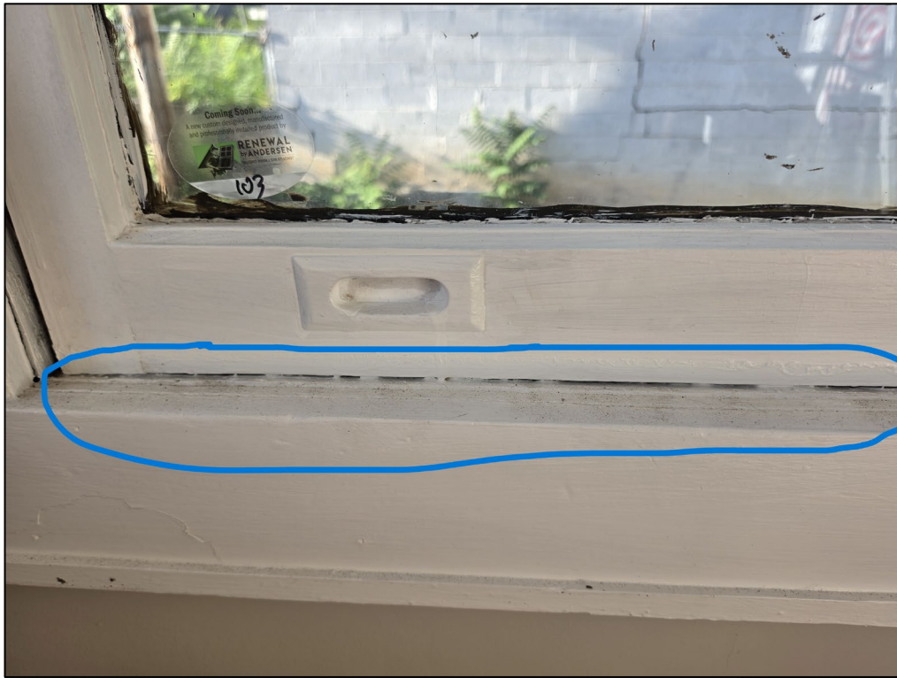
Downstairs bathroom, interior
