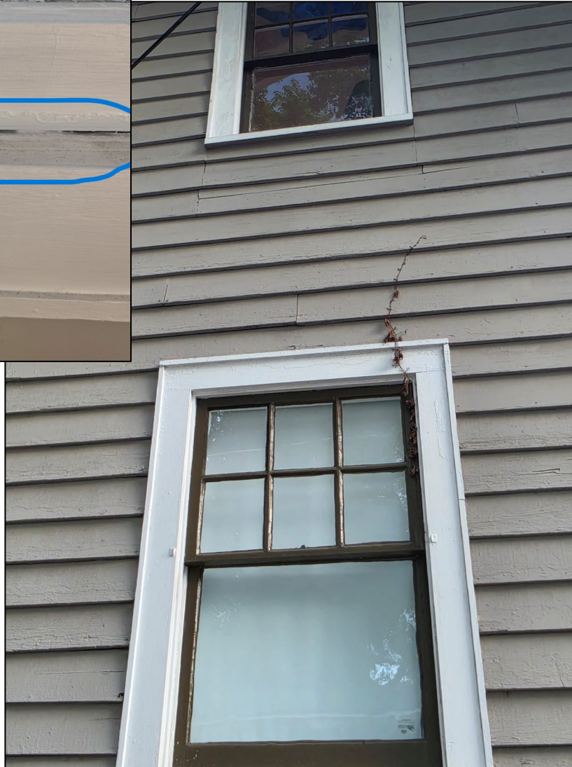
Downstairs bathroom, exterior
