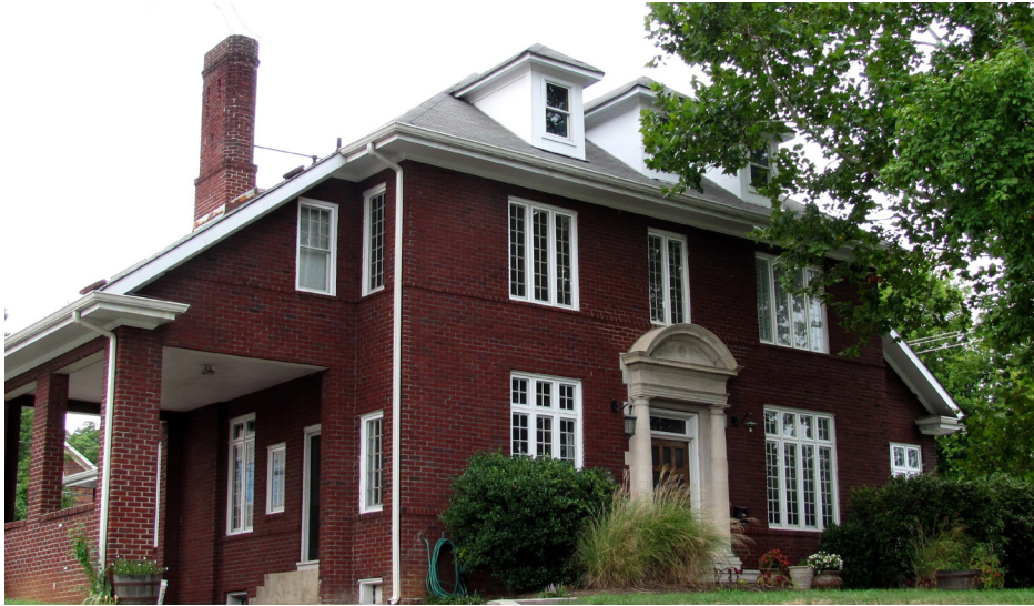
1803 Clinch Ave. Front Facade
