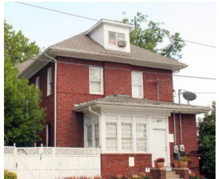
1803 Clinch Ave. Rear Facade
