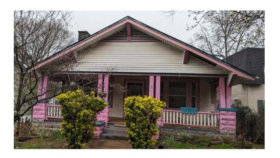
Roofing is beyond its life and is letting water into the house. Requesting approval to have the roofing replaced with architectural asphalt shingles.
