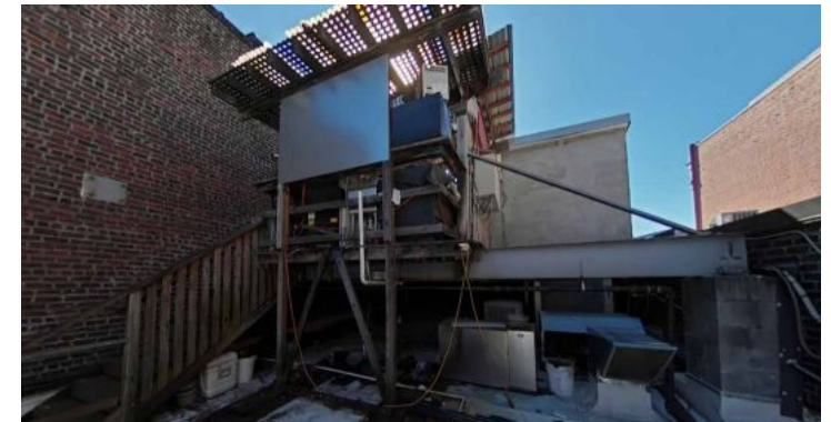
EXISTING ROOF DECK STRUCTURE TO REMAIN; BAR AND TRELLIS TO BE REMOVED. ALL MECHANICAL TO REMAIN AS NEEDED. EXISTING STAIR AND WALKWAY FROM DECK TO BE REPAIRED/REPLACED AS NEEDED
