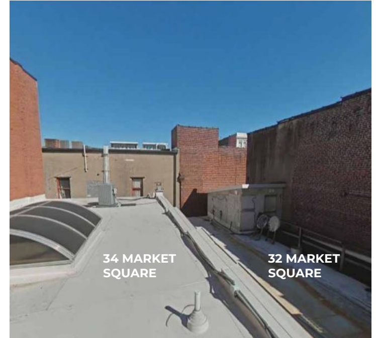
EXISTING ROOF, SKYLIGHTS, AND MECHANICAL EQUIPMENT AT 34 MARKET SQUARE TO BE REMOVED. EGRESS STAIR AT ALLEY SIDE OF 32 MARKET SQUARE TO REMAIN TO BE UTILIZED AS PART OF NEW EGRESS SYSTEM.
