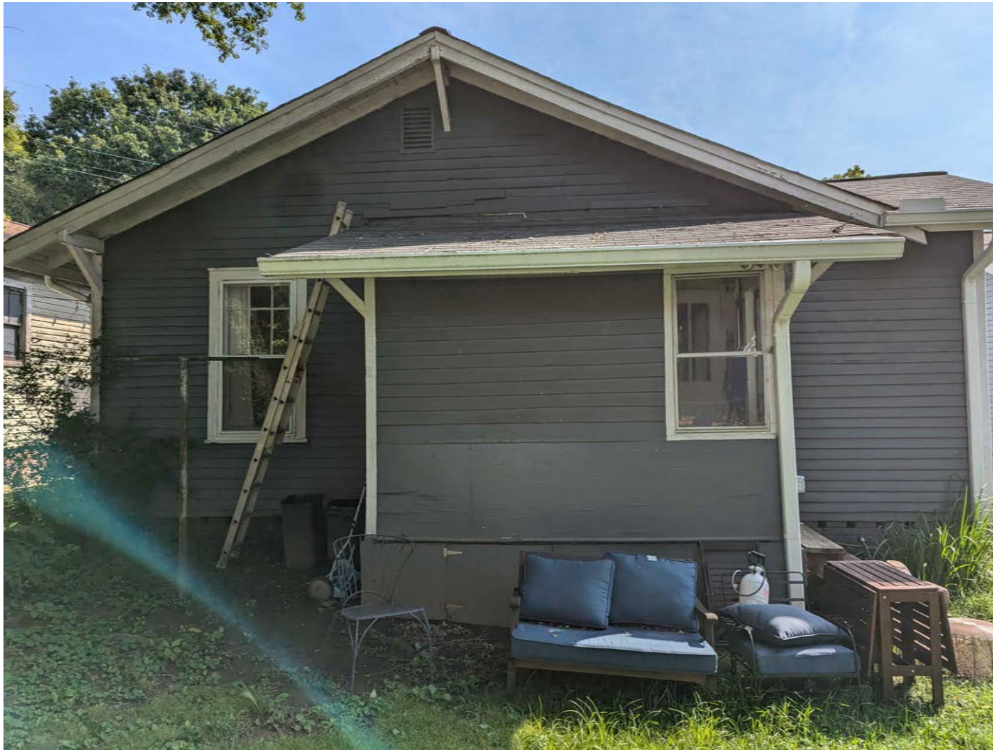
CONNALLY RESIDENCE: EXISTING CONDITION existing rear elevation
