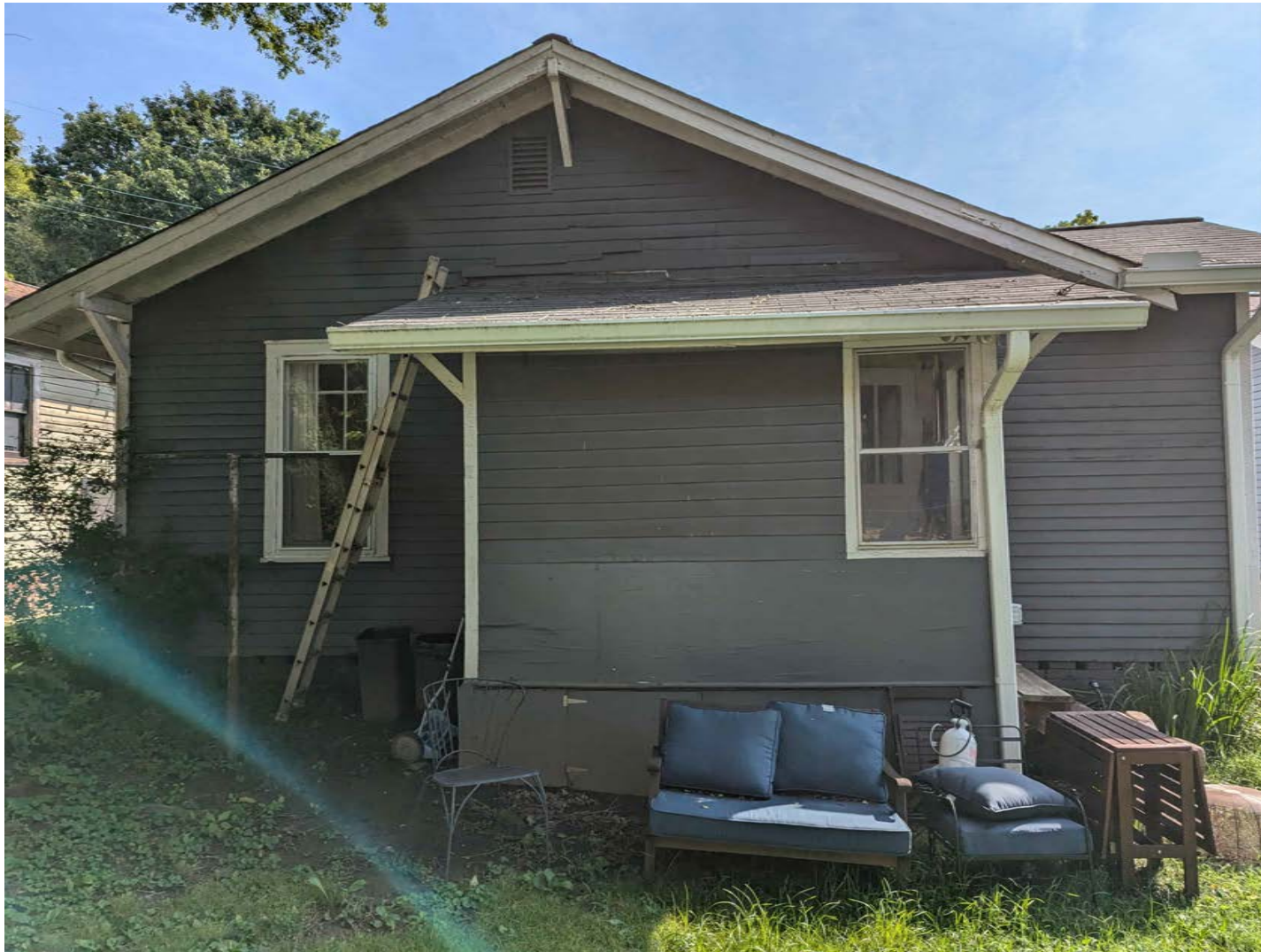
CONNALLY RESIDENCE: EXISTING CONDITION existing rear elevation
