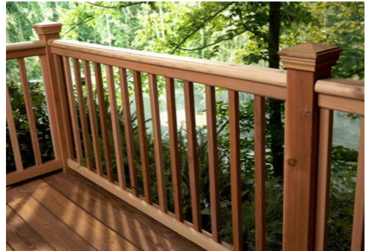
EXAMPLE OF SIMILAR RAILING
