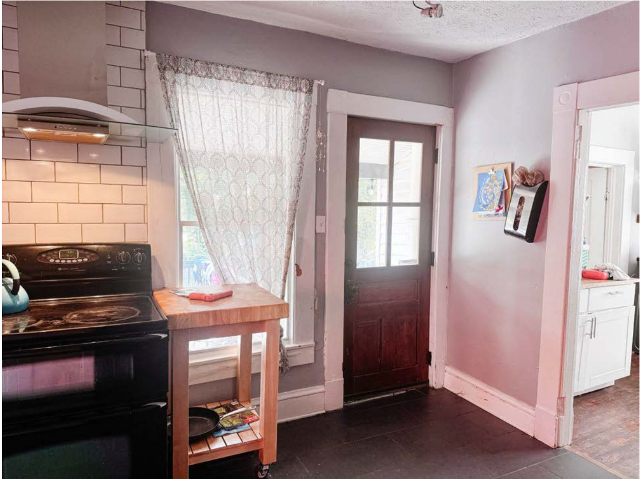
Window to be removed and replaced with existing rear door.
