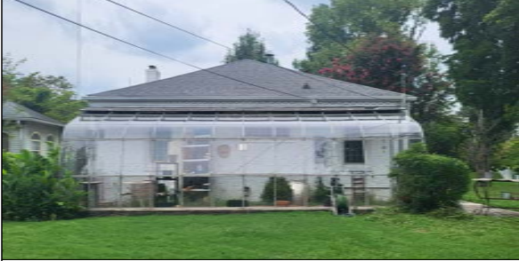
3 EXISTING EXTERIOR PHOTO AD-101
