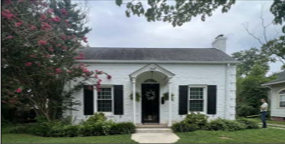
4 EXISTING EXTERIOR PHOTO AD-101
