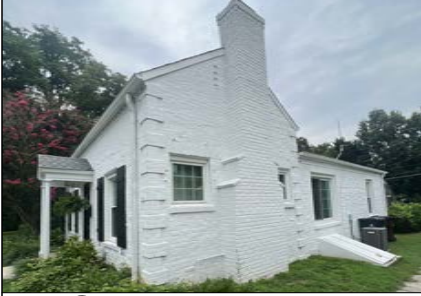
2 EXISTING EXTERIOR PHOTO AD-101
