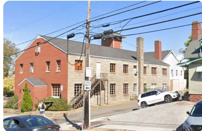
Original Chapel South Elevation
