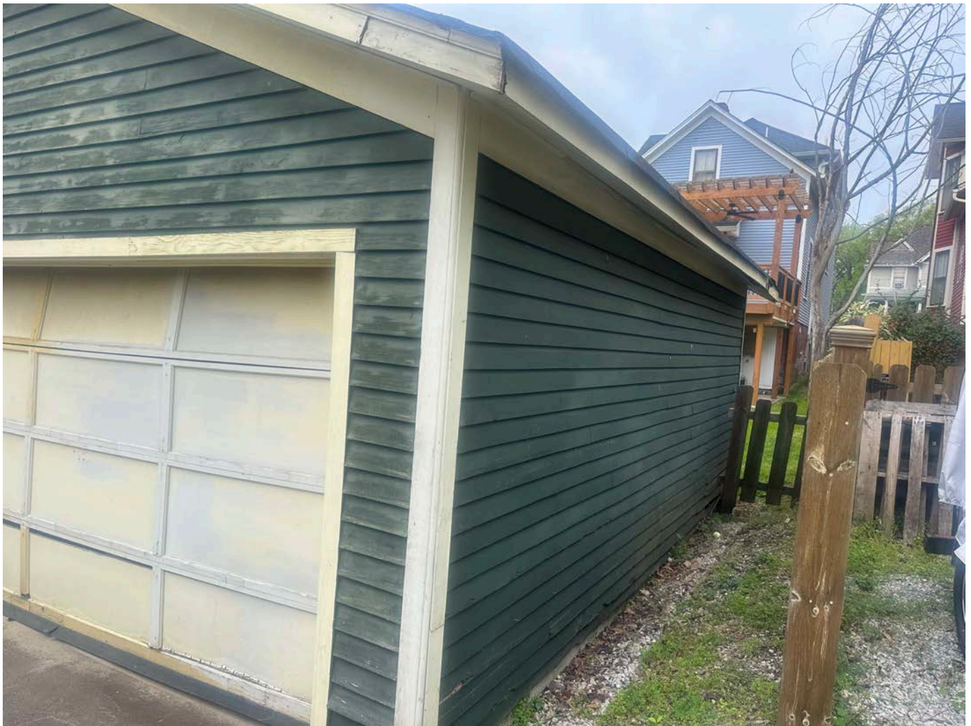
Nothing added just some siding repair on back right corner.
