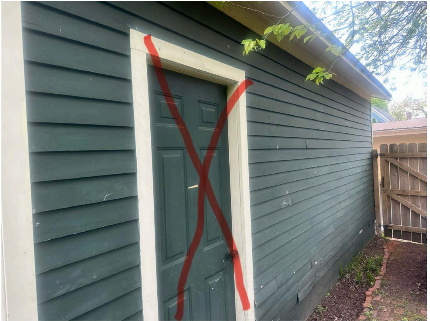
Remove door and frame to install matching siding.
