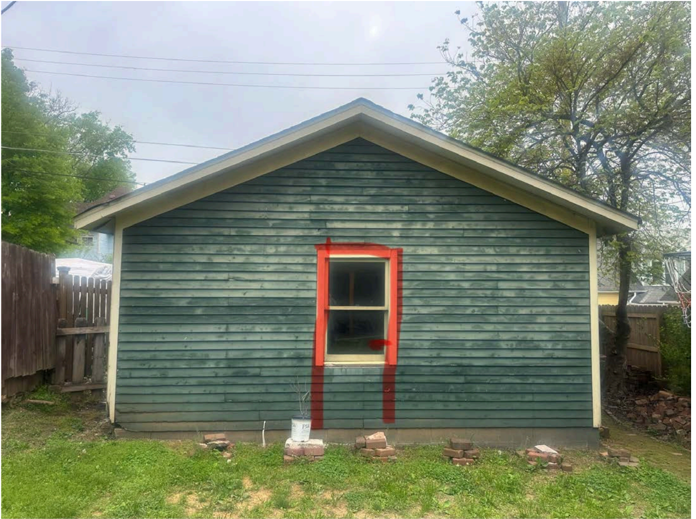
Remove window and install door.
