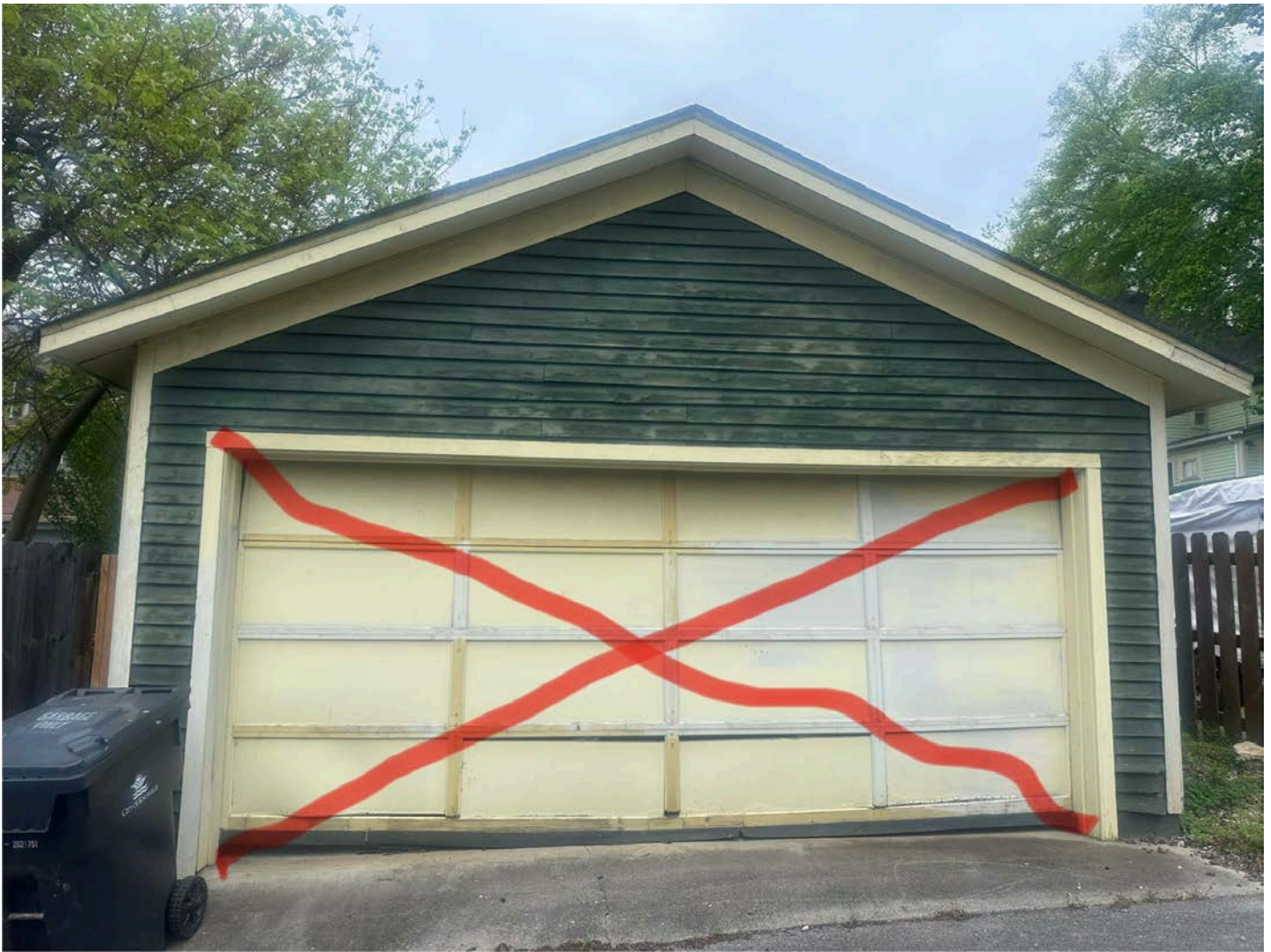
Remove garage door and frame to install matching siding.
