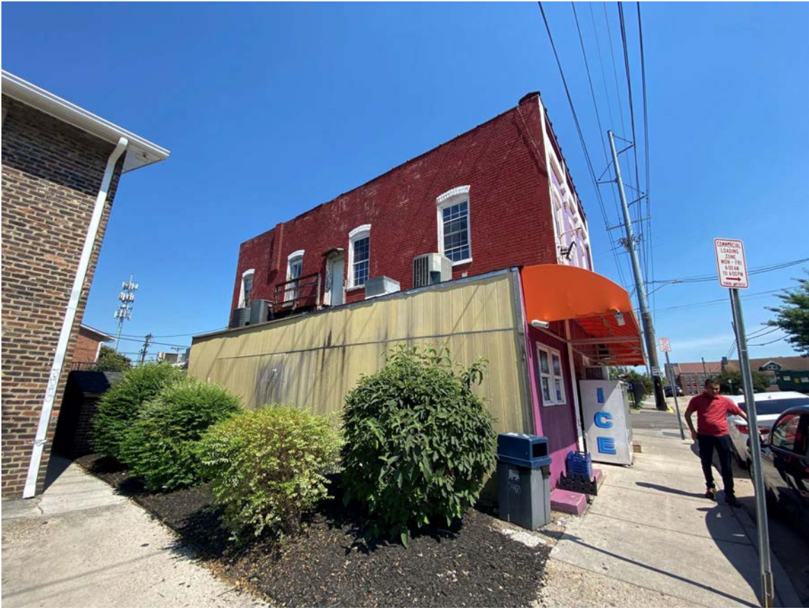
View from 13th St. entering the pool area behind the building.
