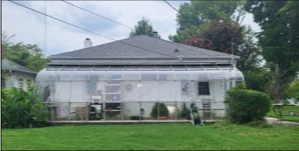
3 EXISTING EXTERIOR PHOTO AD-101
