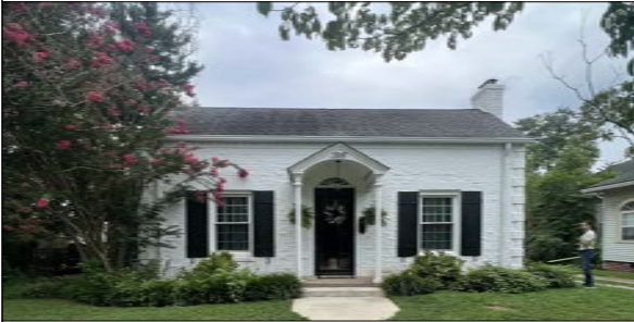
4 EXISTING EXTERIOR PHOTO AD-101
