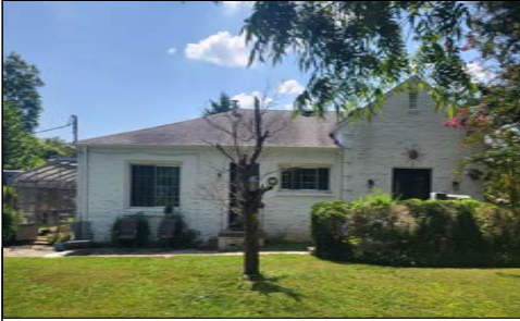
5 EXISTING EXTERIOR PHOTO AD-101
