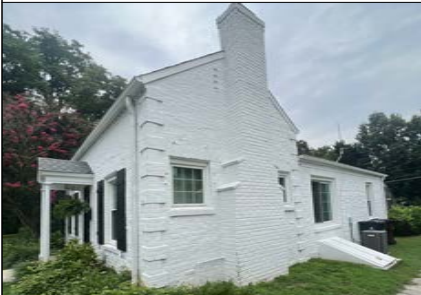
2 EXISTING EXTERIOR PHOTO AD-101
