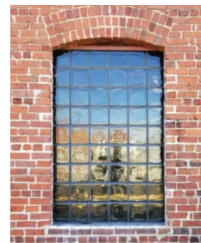
GLASS BLOCK INSTALLED
