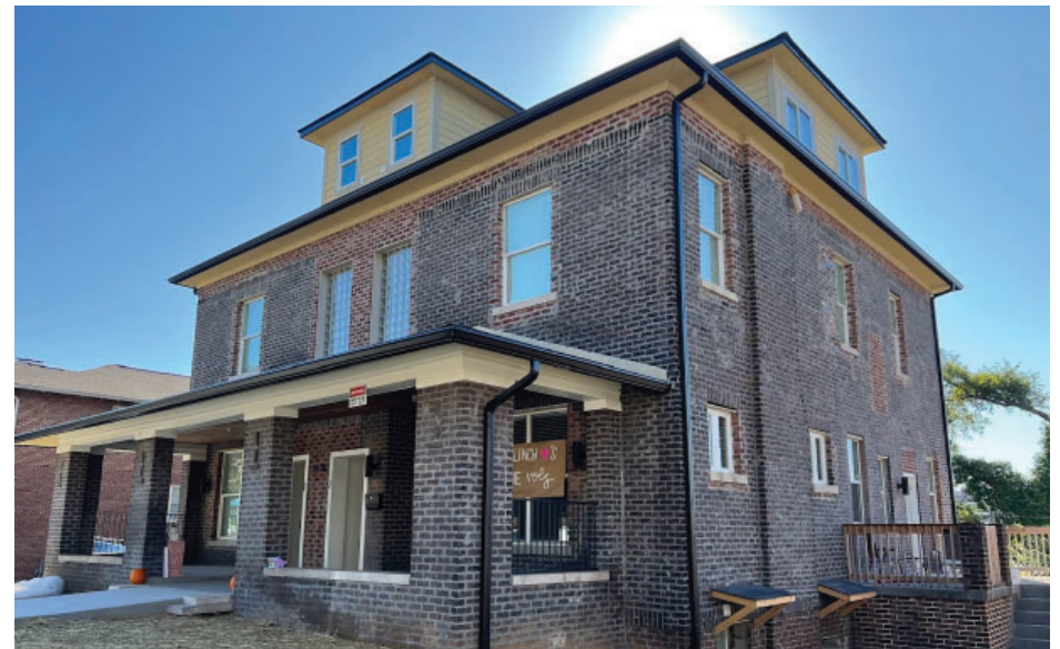
CHANGED/BUILT CONDITION, GLASS BLOCK USED IN 2ND STORY WINDOWS
