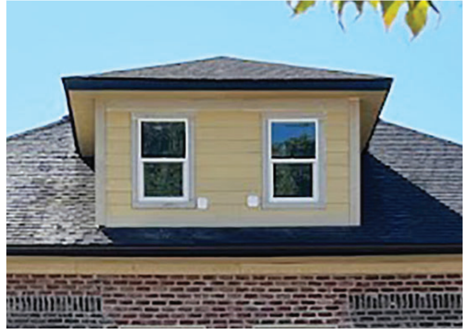
NEW WINDOWS W/ OPAQUE, FIRE RESISTANT BACKING. (TRIM AND SIDING NOT PAINTED AT TIME OF PHOTOGRAPH)
