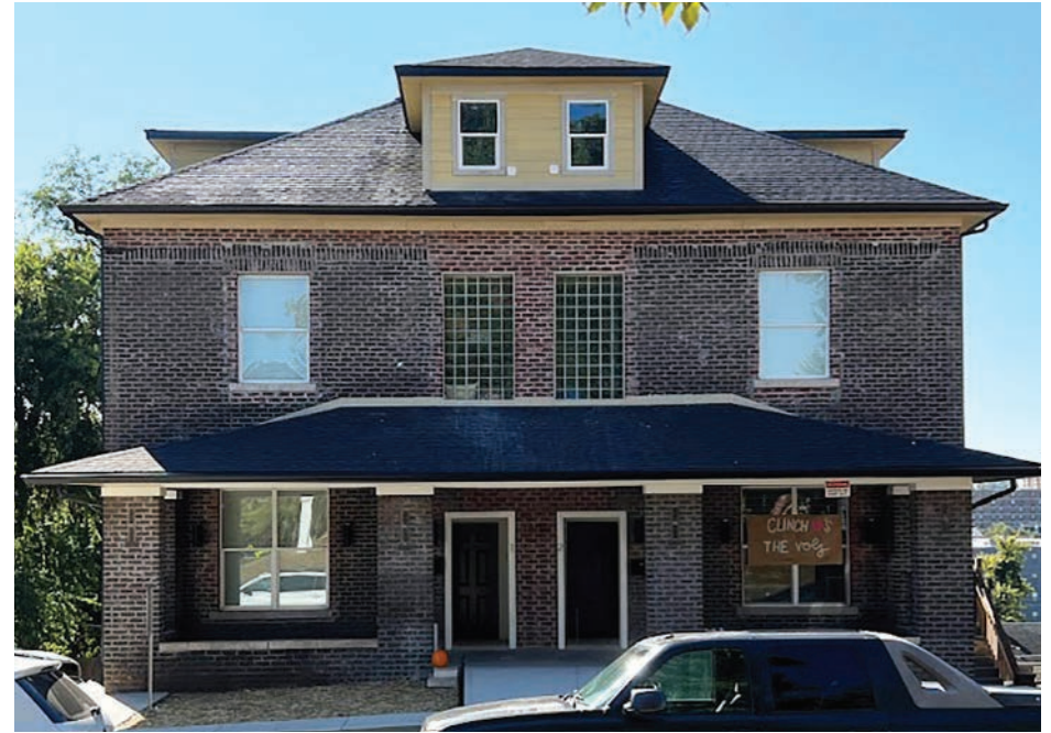
CHANGED/BUILT CONDITION, GLASS BLOCK USED IN 2ND STORY WINDOWS
