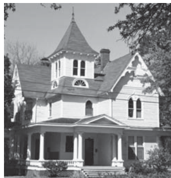
The tower on this Lake Charles Victorian residence is an important part of its design. Were it to be lost, the home’s National Register design integrity would be severely compromised.
