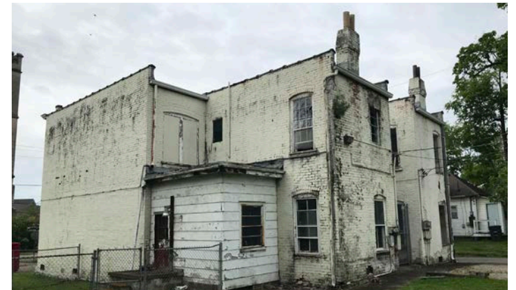
EXISTING BRICKWORK TO BE REPAIRED AND REPAINTED IN KIND TO MAINTAIN HISTORIC CHARACTER
