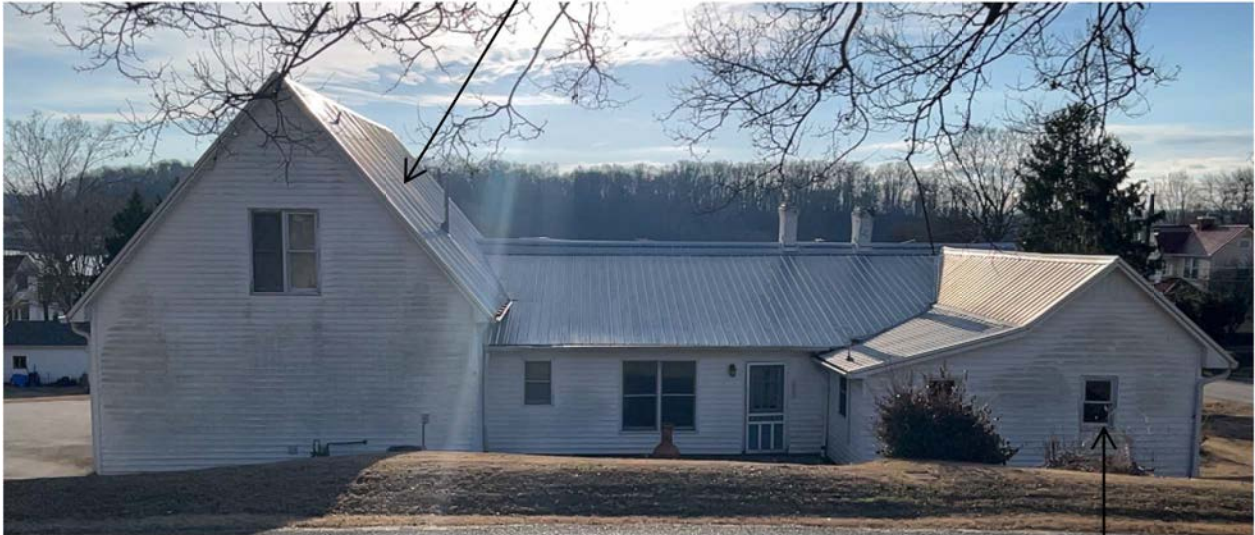
Elevation facing North
