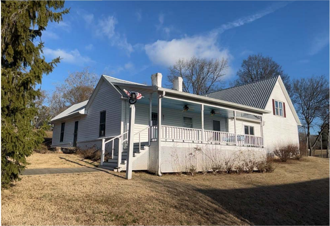
1000 Olive Road; View facing North
