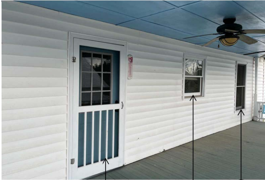
Existing Porch Elevation Facing South
