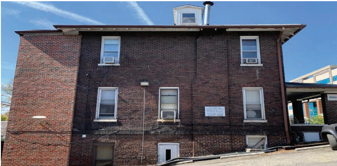
EXISTING WINDOWS TO BE REPLACED WITH SHORTER WINDOWS TO ACCOMMODATE NEW KITCHEN ON THE INTERIOR
