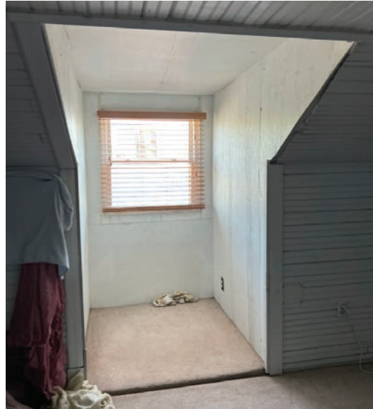
EXISTING ROOF TO BE REBUILT TO PROVIDE 8' CEILING ON THIRD FLOOR
