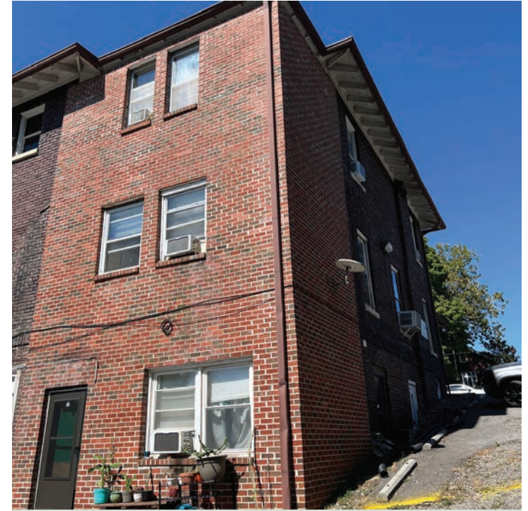
REPOINT BRICK WALLS AS NEEDED AND SEAL BRICK WALLS AND JOINT BETWEEN BRICK AND PAVEMENT
