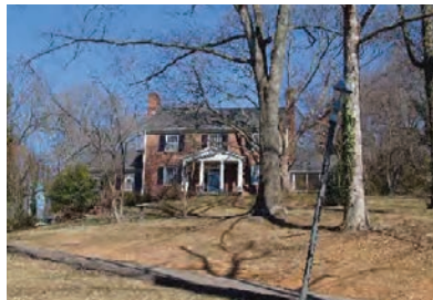
800 Blows Ferry Road
