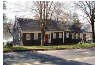
805 Blows Ferry Road
