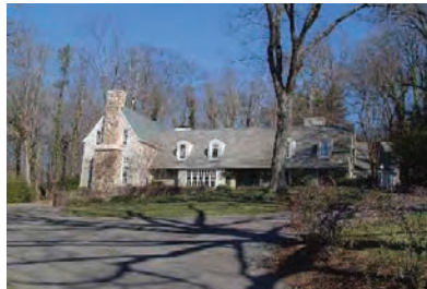
710 Blows Ferry Road
