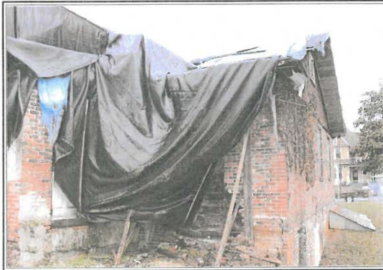
Southeast Corner of Building
