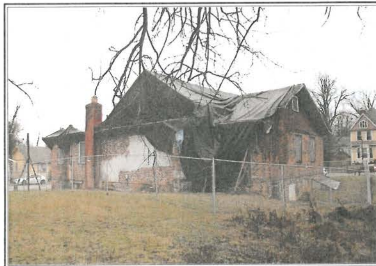
Rear View & East Side
