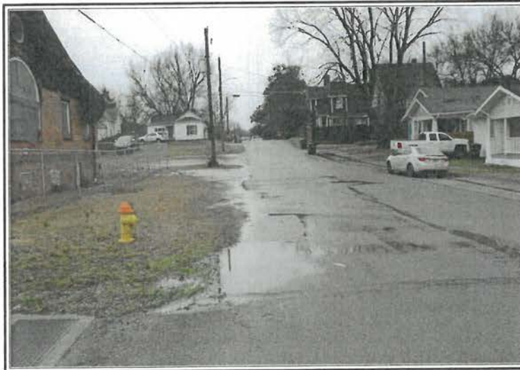
View Along Polk Street - Subject on Left
