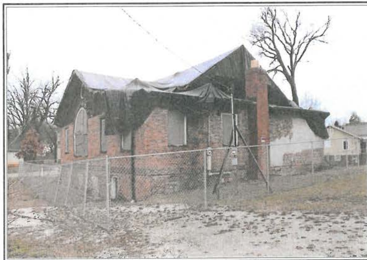
West Side & Rear View
