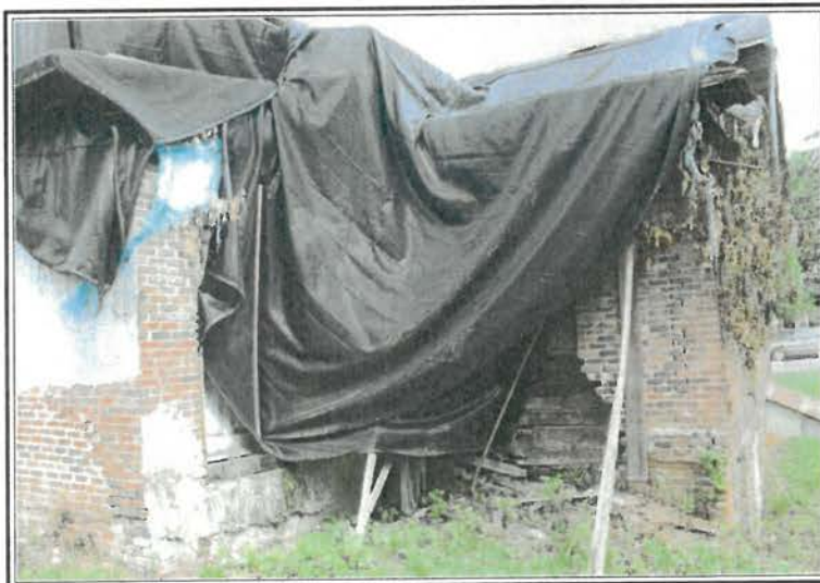
Rear Southeast Corner
