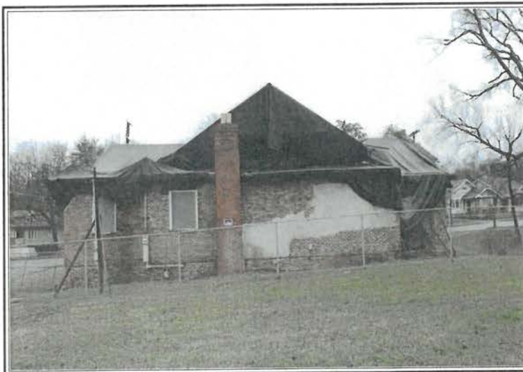
REAR OF SUBJECT PROPERTY
