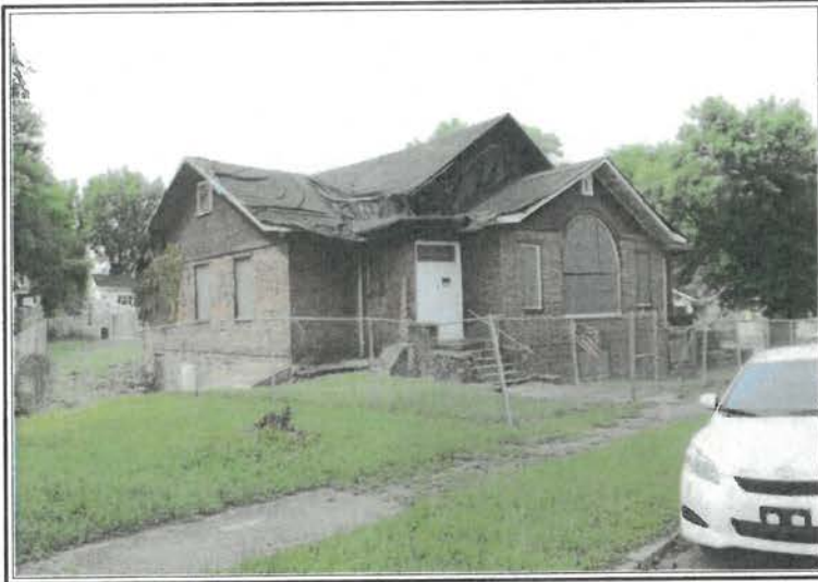
Front View and East Side
