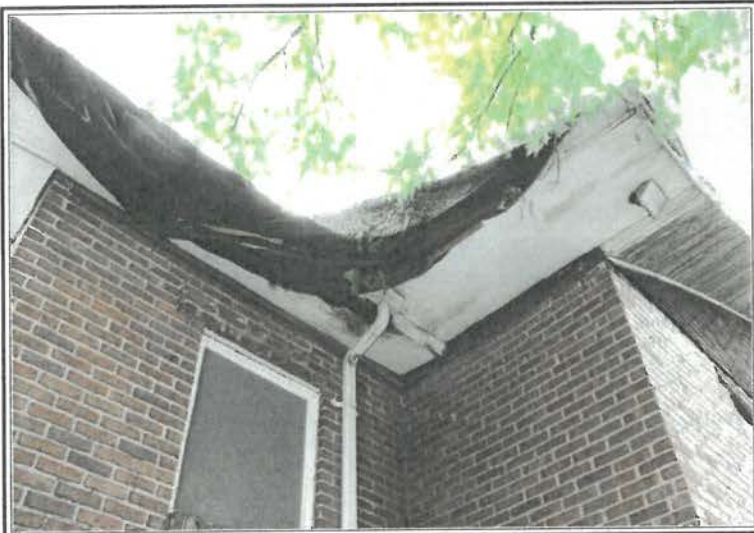
Front West Side Eave
