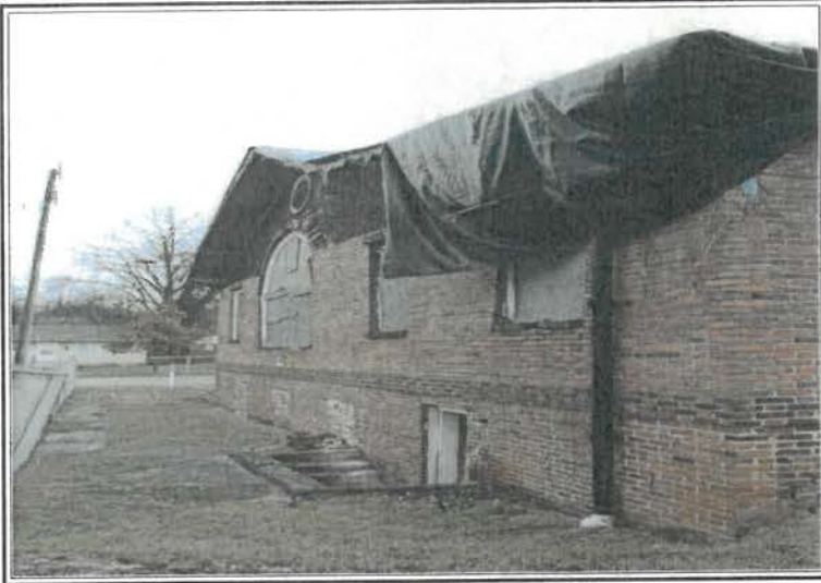
West Side with access to basement
