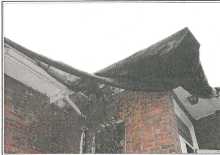
Northeast Corner of Building
