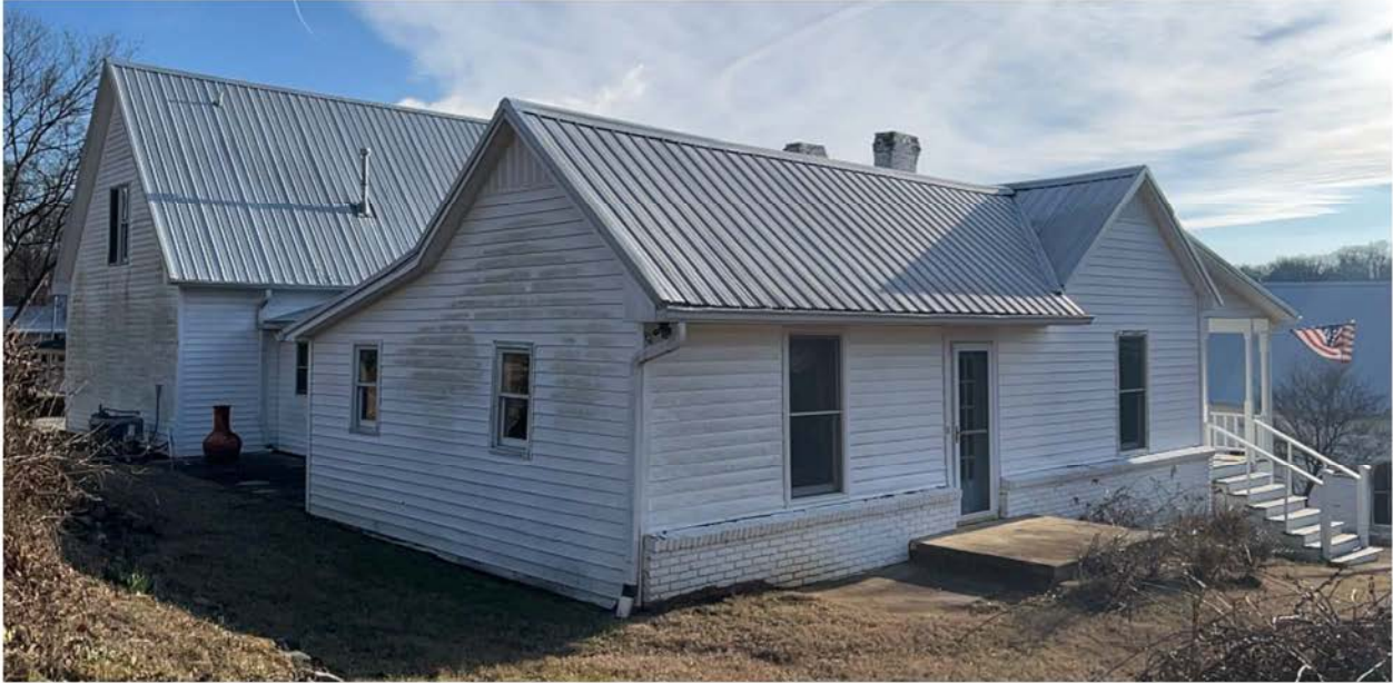
View facing East
