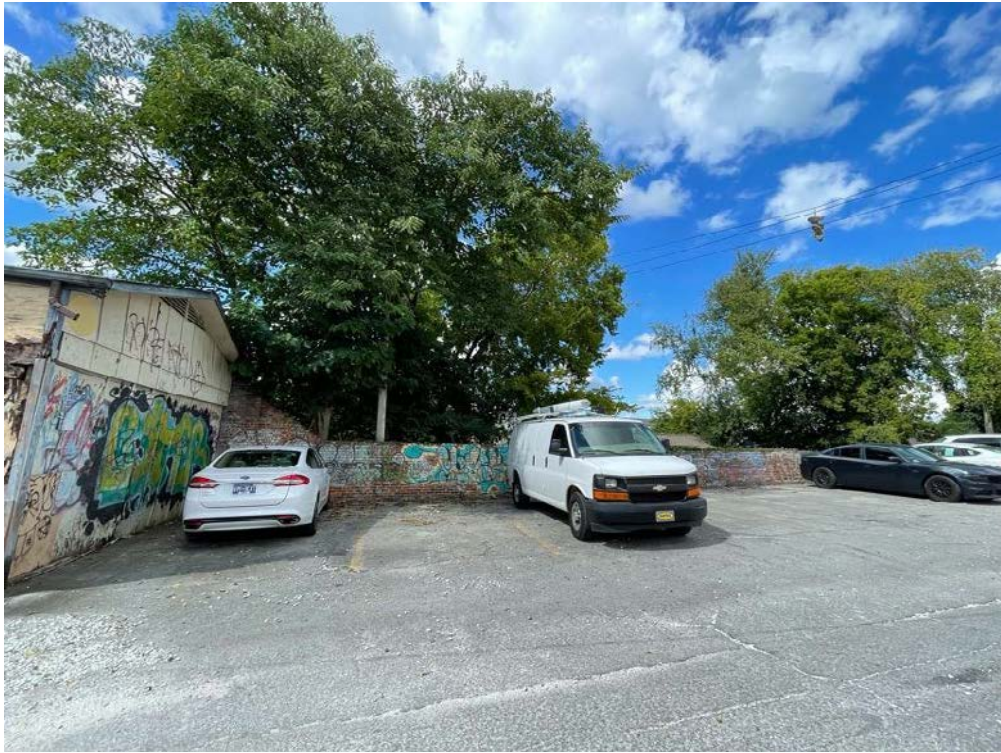
Building and retaining wall, facing north
