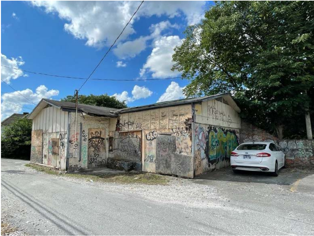
Building, facing northwest
