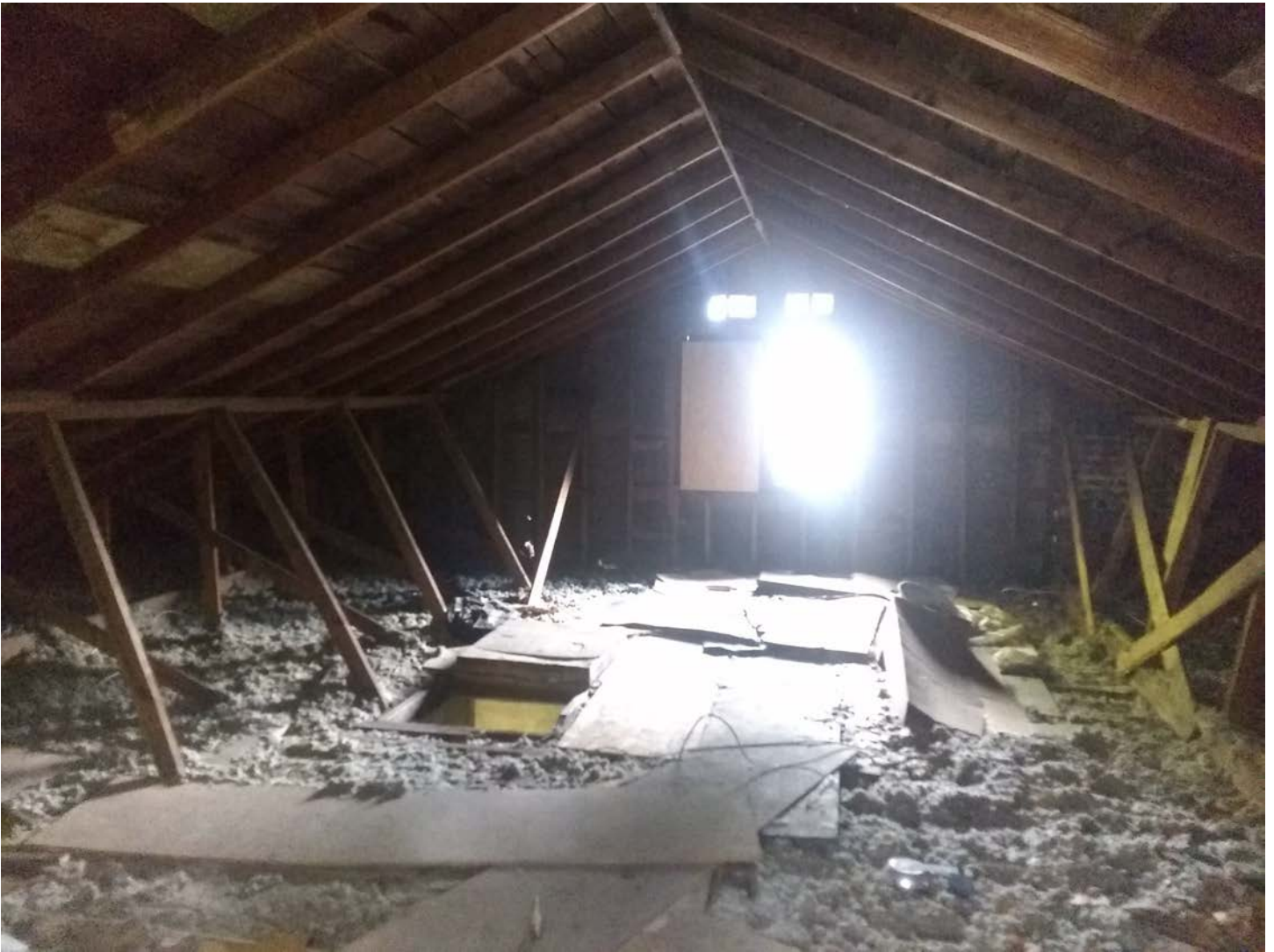
Facing south. Note: left window is removed and covered. This is being used as the template for the replacement to be installed on the north side.
