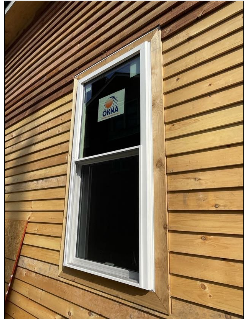
Window and trim detail photo taken by staff
