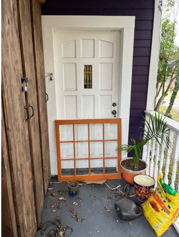
The refurbished window.
