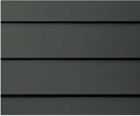
FIBER CEMENT LAP SIDING, TYPICAL
