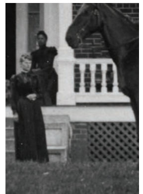
ORIGINAL EXTERIOR RAILING
