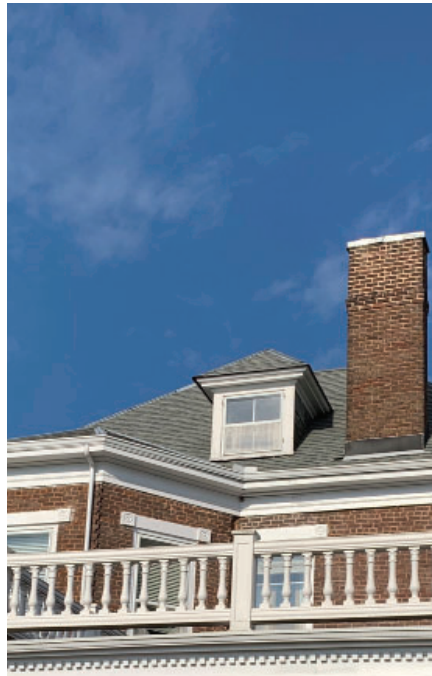
CHIMNEY (SW) - CURRENT
