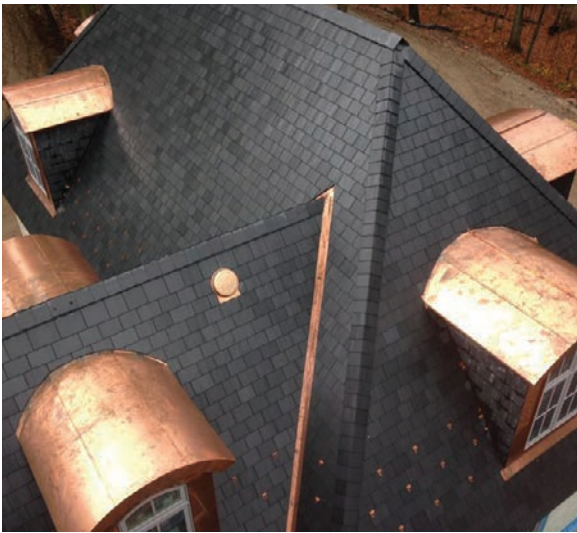
PROPOSED BLACK SLATE AND COPPER SNOW CLEATS
