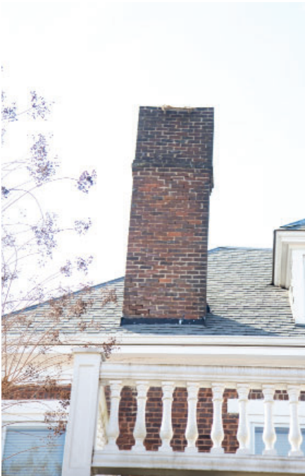
CHIMNEY (SE) - CURRENT
