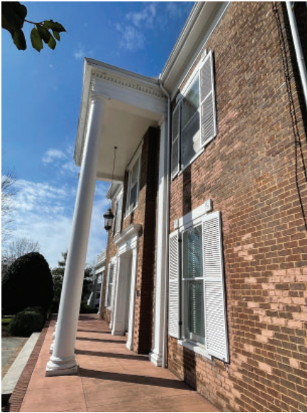
REMOVE PAINT OFF BRICK WALLS THROUGH DRY ICE BLASTING
