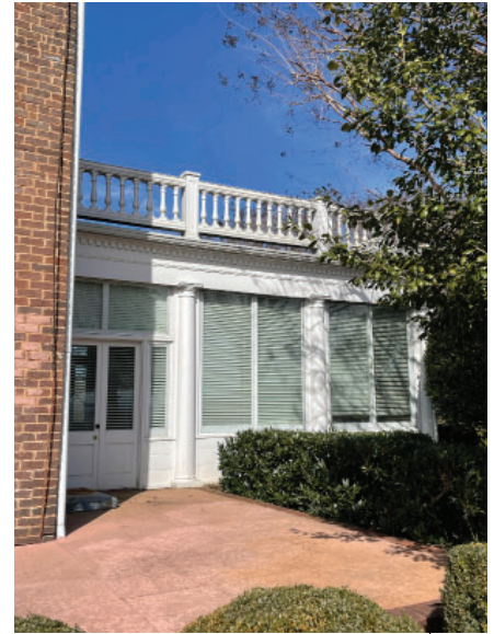
REMOVE ALL INTERIOR PARTITION WALLS, EXTERIOR ENVELOPE, AND REOPEN TO A COVERED PORCH WITH TENNESSEE MARBLE PAVERS - REFER TO PAGE # 17
