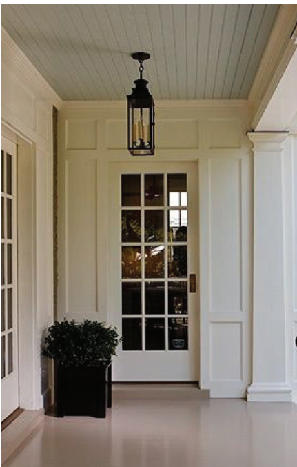
PROPOSED WOOD BEADBOARD CEILINGS - TYPICAL ALL PORCHES AND SUNROOMS
