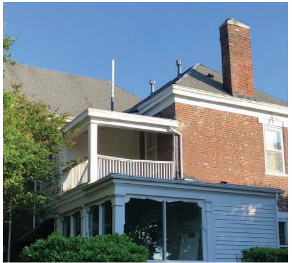
EXISTING BALCONY WALL WITHOUT ACCESS DOOR
