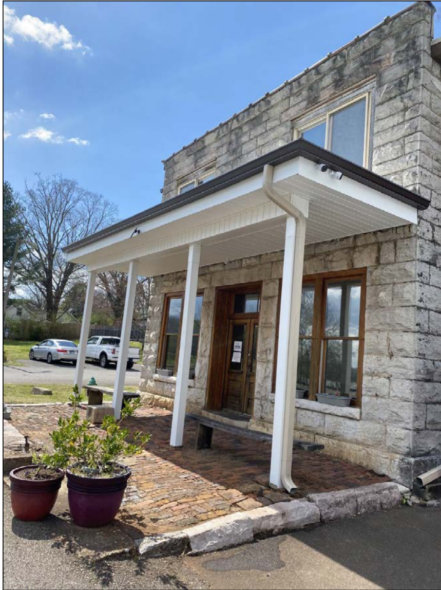
Photo of work completed, submitted by contractor
