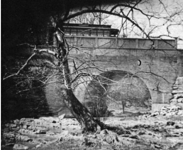
Trolley + Broadway bridge at First Creek, early 20th century
