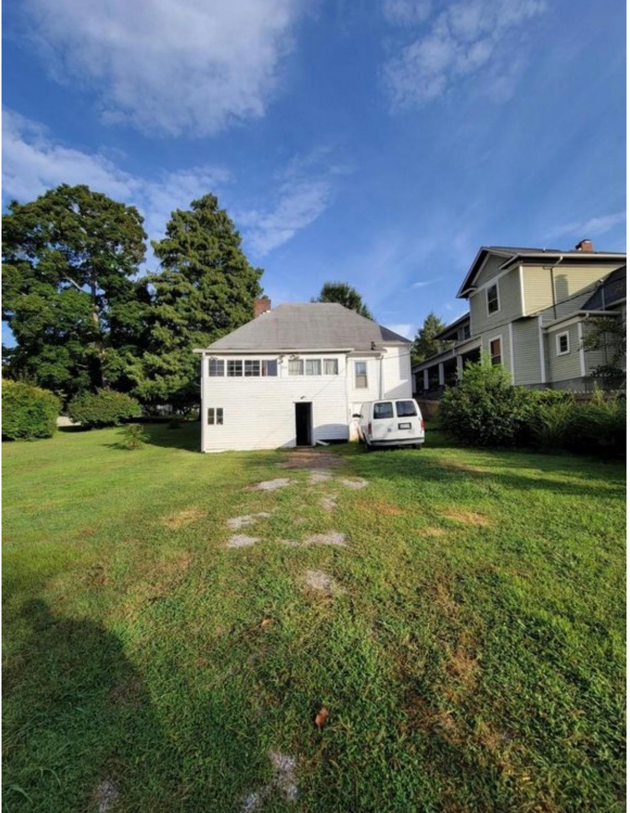
Here is a photo of the changes that have been made to the siding:
