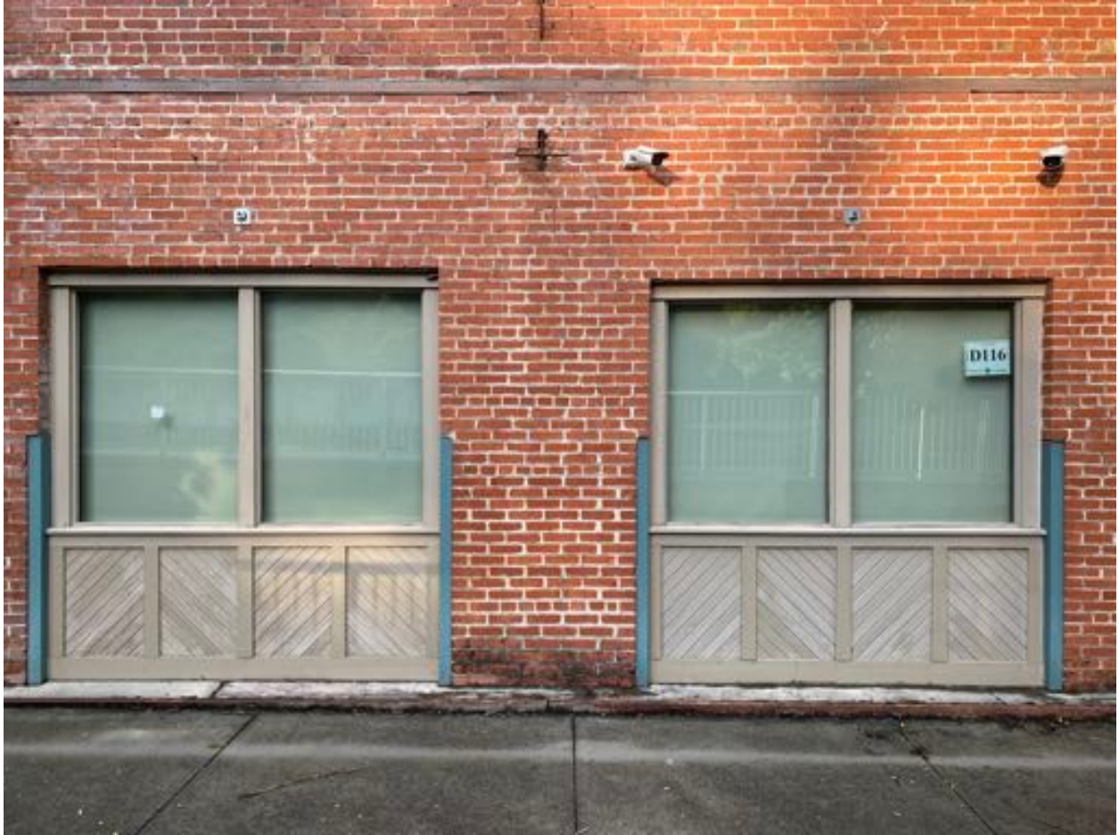
L&N Freight Depot - Inspiration for panels.
