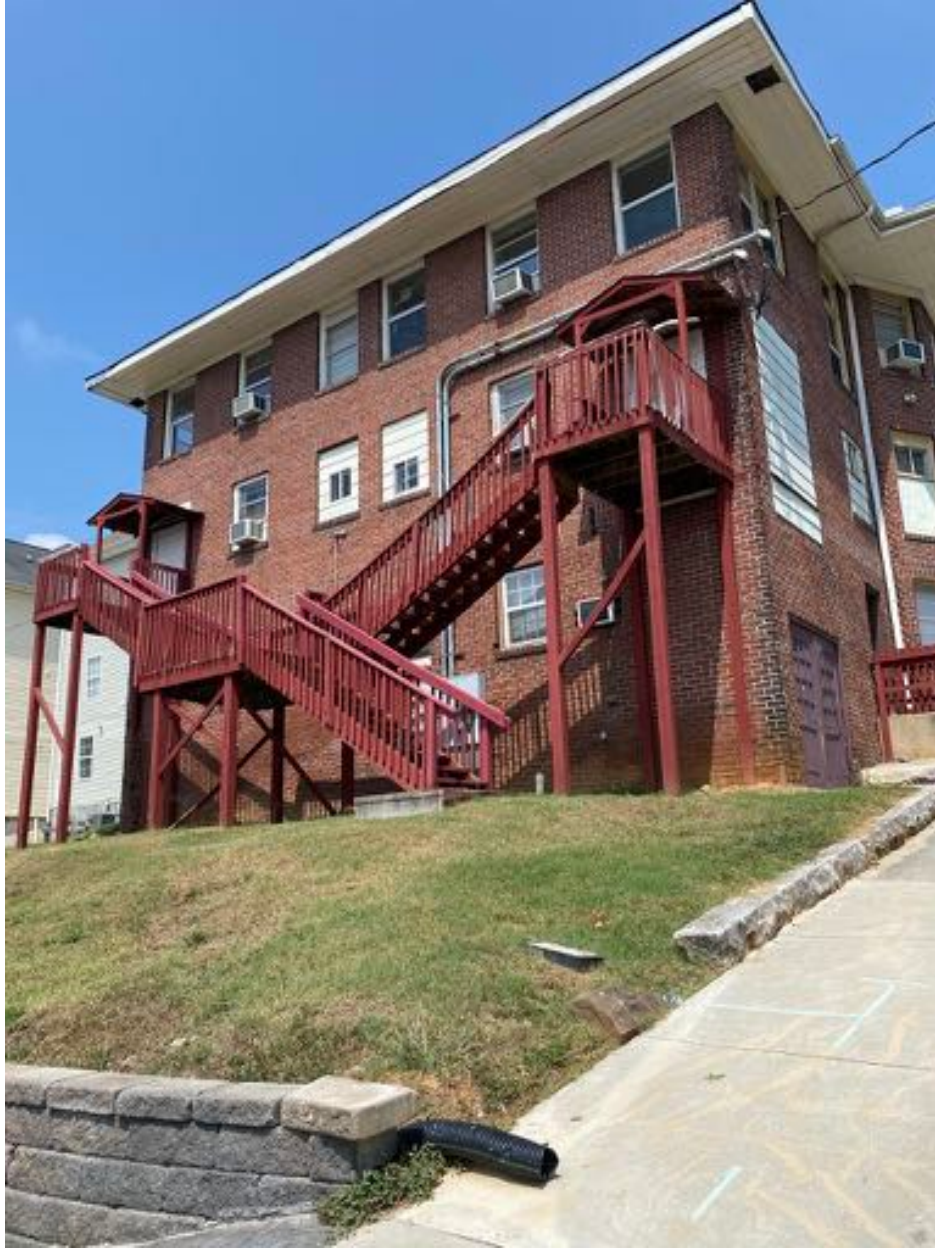
Existing Conditions - Rear, 12th Street Shows Existing Exterior Stairwell that is to remain and be evaluated for maintenance and repair.
