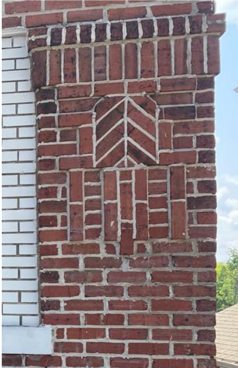
Existing Conditions - Brick Detail on porch piers and front chimneys.
