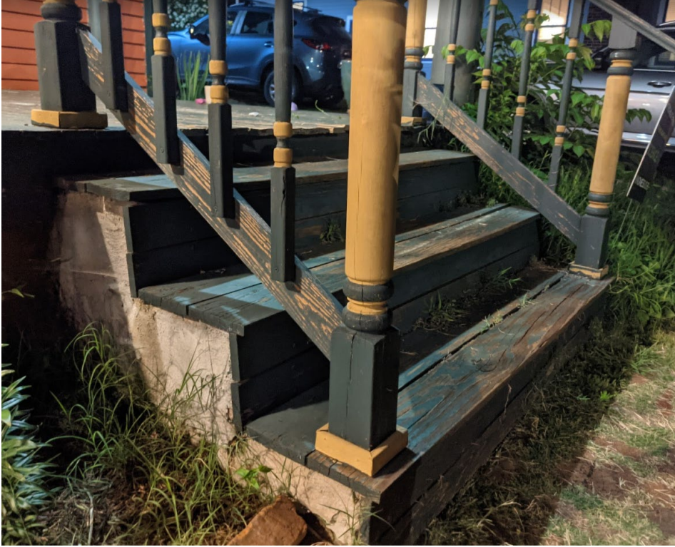
Wood overlay on concrete steps and improperly secured handrails
