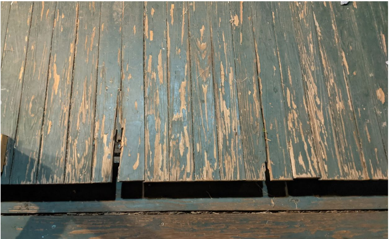
Deterioration of decking.
