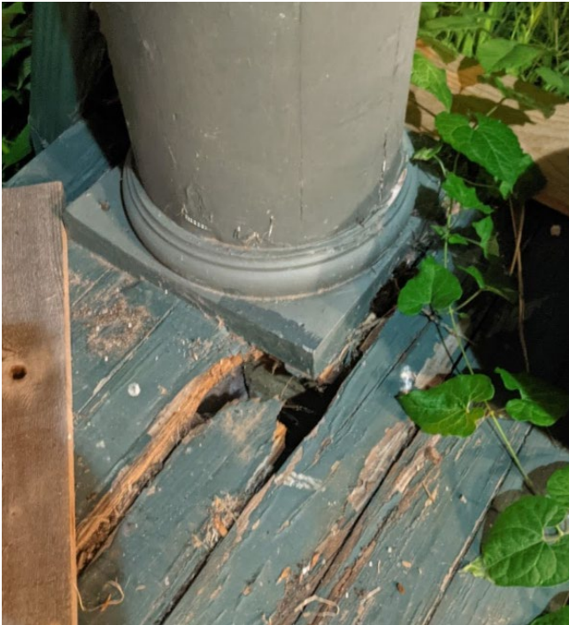
Decomposition of decking around eastern most column, rear side of column
