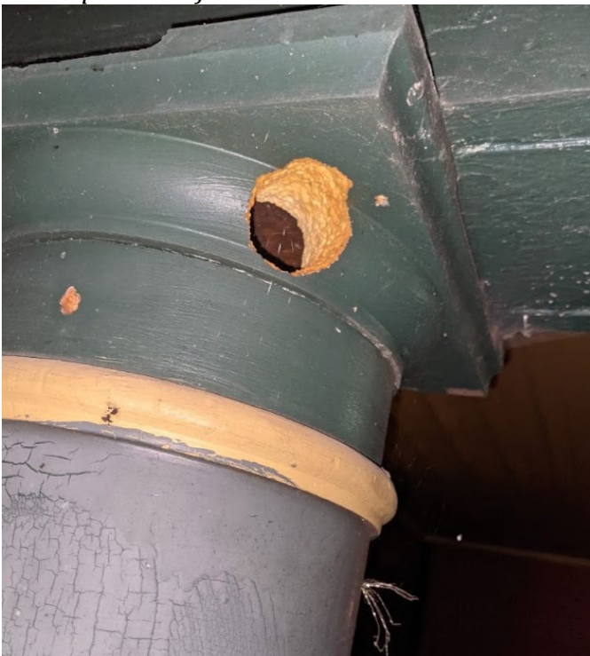
Example of bird damage to top cap of columns (Representative of damage on all 4 columns)
