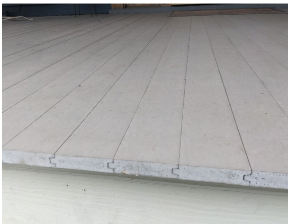
Proposed T&G Porch Flooring, installed in neighborhood property.
