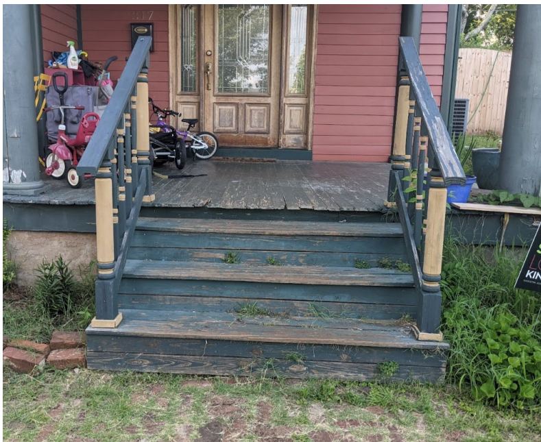
Deteriorated wood overlay on concrete steps
