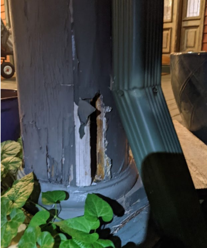
Decomposition of eastern most column due to combination of weather and animal nesting.
