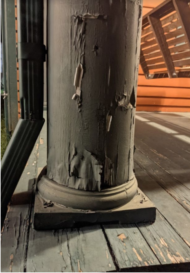
Rot damage of western most column.
