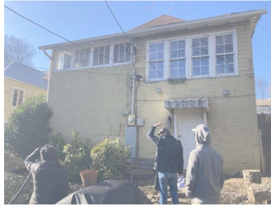
322 EAST OKLAHOMA - EXISTING REAR ELEVATION NEW/EXTENDED ROOF LINE NOT VISIBLE
