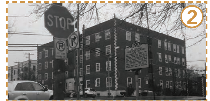
^ Shows roof and material precedent.
