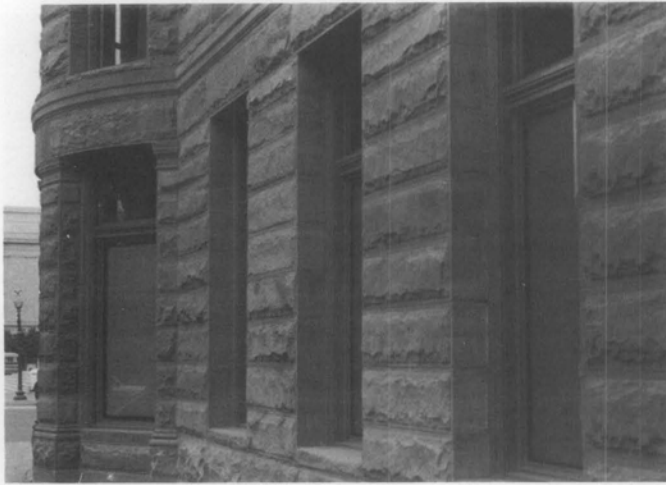
Illus. 16. The good quality substitute materials shown here do match the historic sandstone in color, texture, tooling and surface details. Dry-tamp cast stone was used to match the red sandstone that was no longer available. The reconstructed first floor incorporated both historic and substitute materials. Sufficient molds were made to avoid the problem of detecting the substitutes by their uniformity. Photo: Sharon C. Park, AIA.
