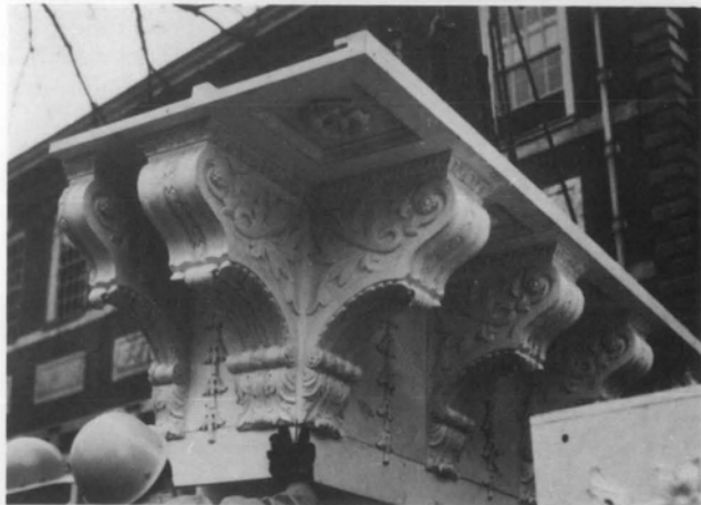
A fiberglass cornice for the reconstruction of an 18th-century wooden clockcase is being lifted in pre-fabricated sections. The level of detail is intricate and of high quality. Photo: Courtesy of Independence National Historical Park.
