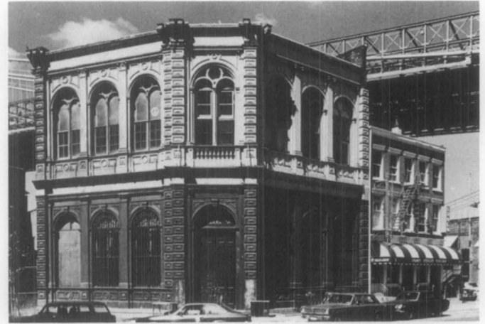
Illus. 4. The 19th-century also produced a variety of metal products used in imitation of other materials. In this case, the entire exterior of the Long Island Safety Deposit Company is cast-iron representing stone. Photo: Becket Logan, Friends of Cast Iron Architecture.
