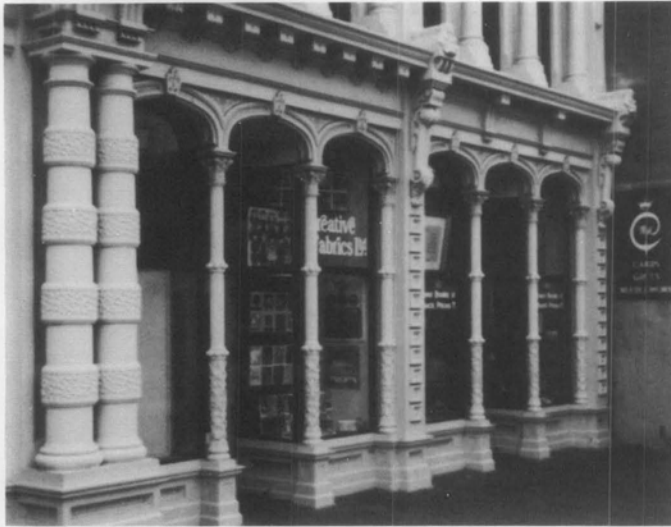
Illus. 11. The unavailability of historic craft techniques is another reason to consider substitute materials. The original first floor cast iron front of the Grand Opera House, Wilmington, DE, was missing; the expeditious reproduction in cast aluminum was possible because artisans working in this medium were available. Photo: John G. Waite.
