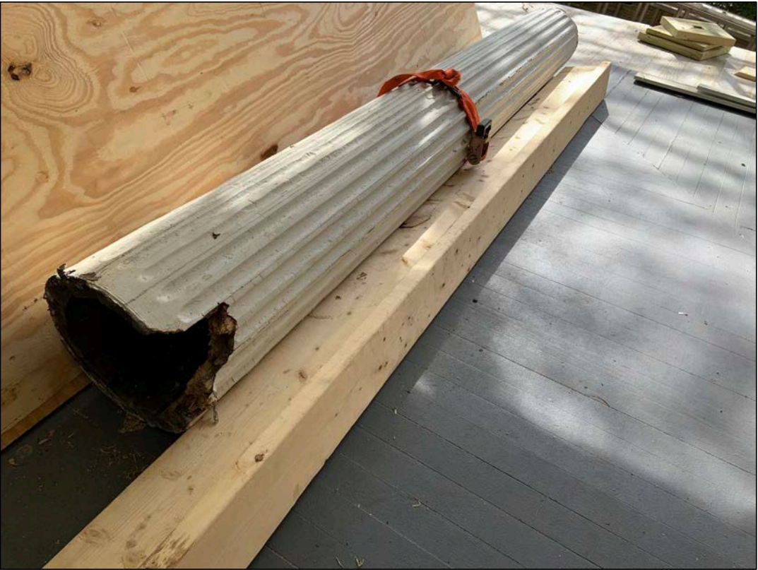
Photo of columns submitted by applicant
