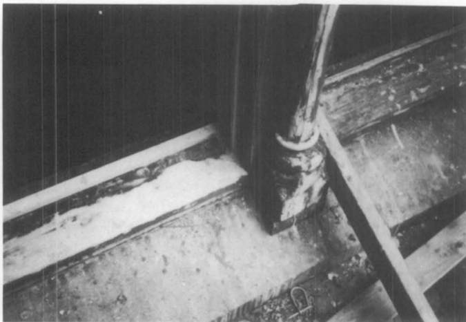
Illus. 7. Whenever possible, historic materials should be repaired rather than replaced. Epoxy, a synthetic resin, has been used to repair the wood window frame and sill at the Auditors Building (1878) Washington, DC. The cured resin is white in this photo and will be primed and painted. Photo: Lee H. Nelson, FAIA.
