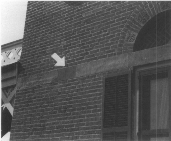
Illus. 21. Change of color over time is one of the greatest problems of synthetic substitute materials used outdoors. Ultra-violet light can cause materials to change color over time; some will lighten and others will darken. In this photograph, the synthetic patching material to the sandstone banding to the left of the window has aged to a darker color. Photos: Sharon C. Park, AIA.
