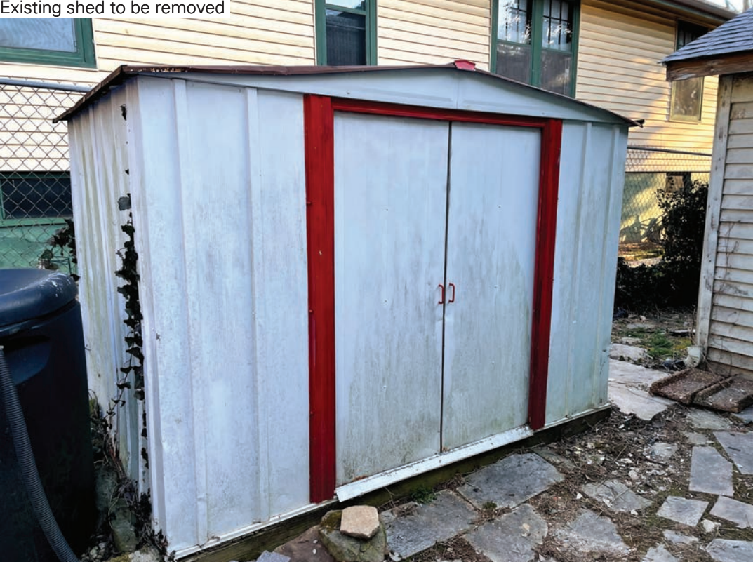
Existing shed to be removed
