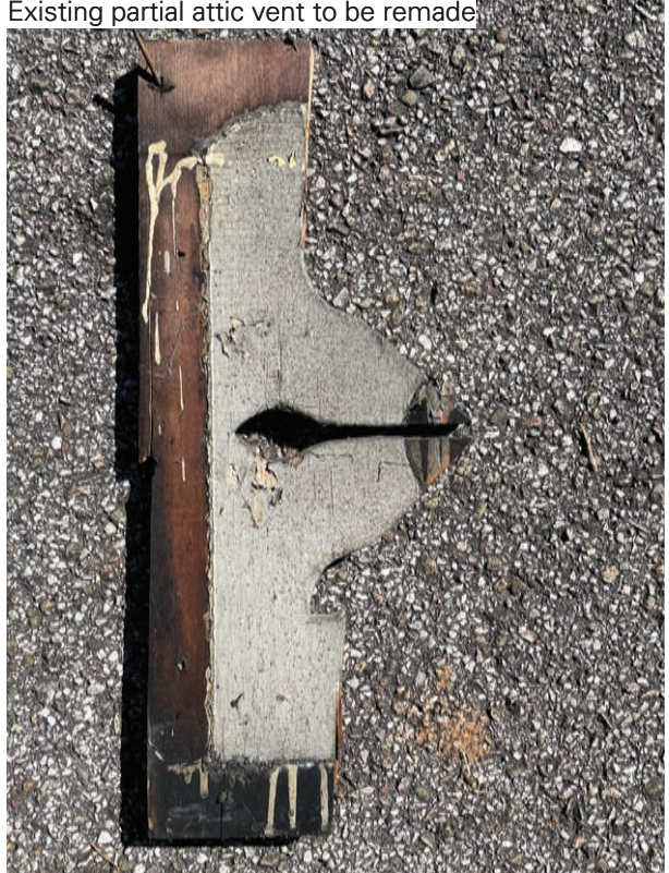
Existing partial attic vent to be remade
