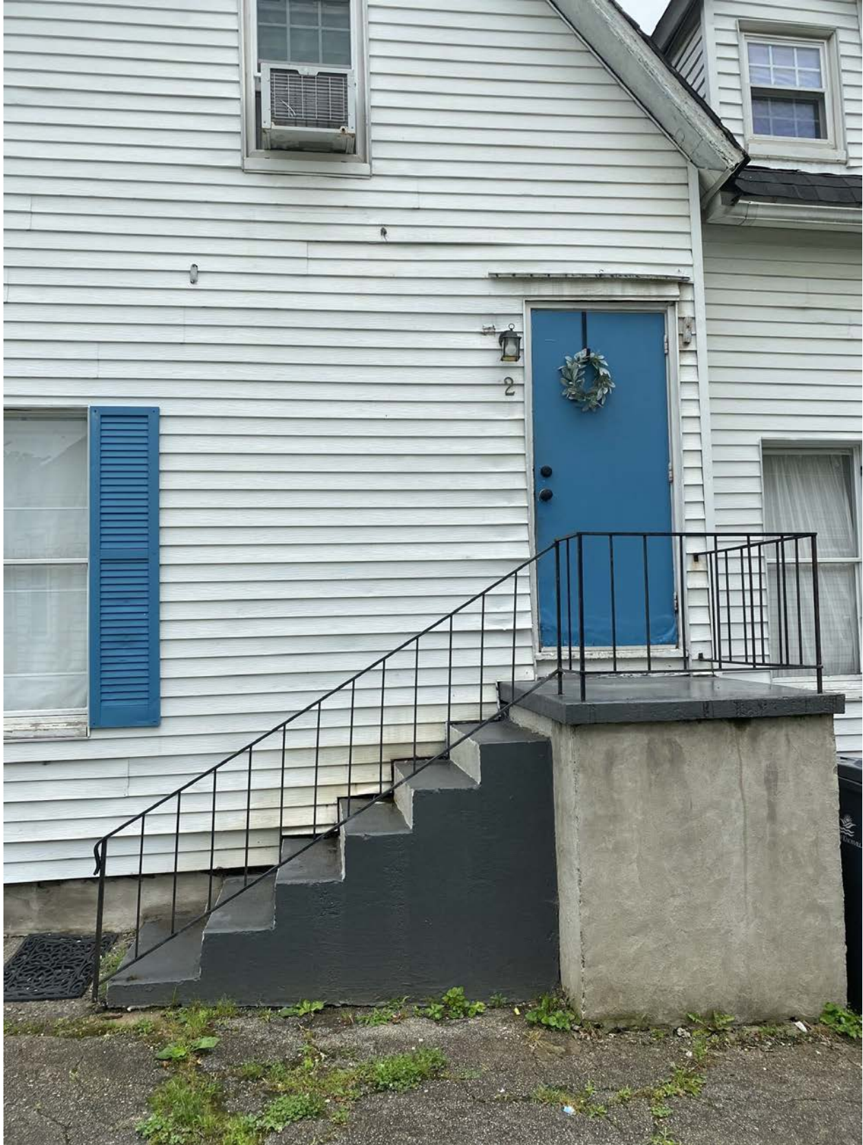
Right side of house with non historic entrance to be demolished.
