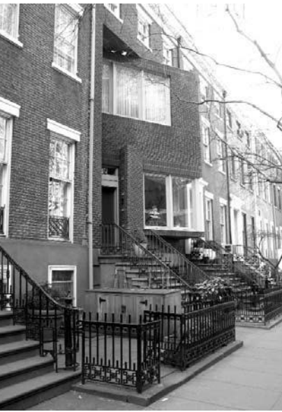
Figure 7. Greenwich Village Townhouse, New York, NY, by Hardy Holtzman Pfeiffer Architects, completed 1978.
