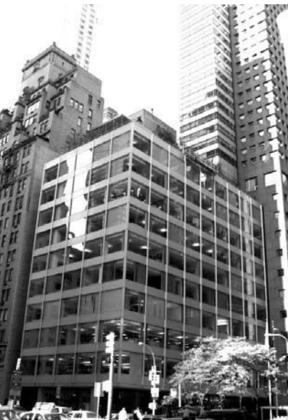
Figure 4. 500 Park Avenue, New York, formerly Pepsico Building (Skidmore, Owings & Merrill, 1960) with office tower addition (right) by James Stewart Polshek and Partners, 1985.
