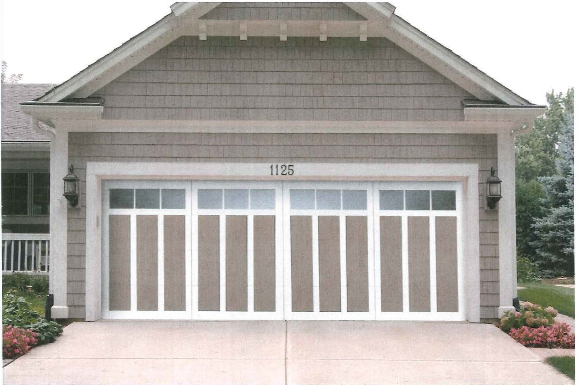
Haas Garage Door Factory, Picture
